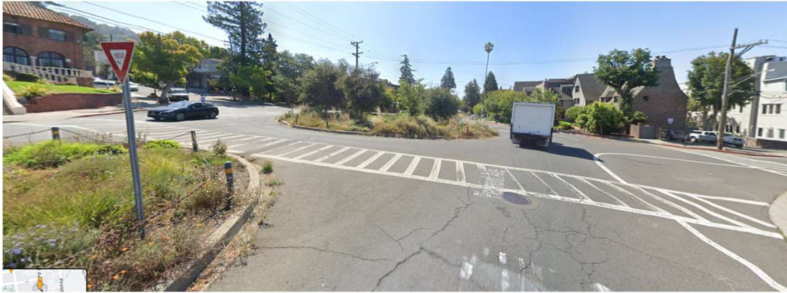
Existing Condition at Piedmont Crosswalk (North)
