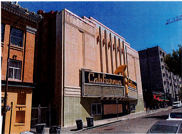
2 STREET VIEW LOOKING NORTH
