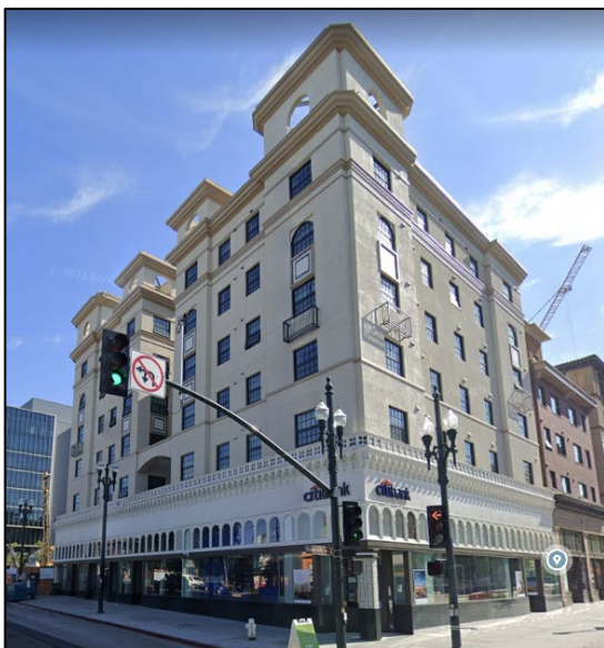
Figure 21: Acheson Commons example (SW Corner)
