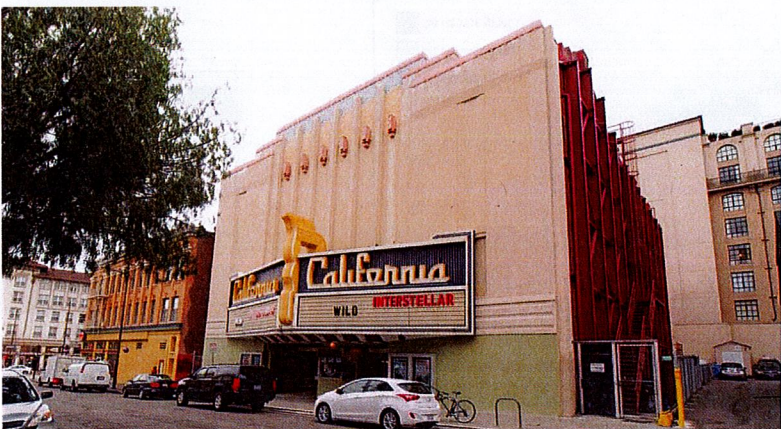
3 STREET VIEW LOOKING WEST
