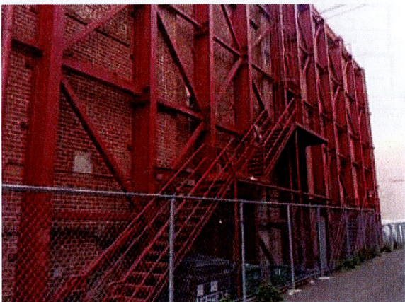
5 EAST SIDEYARD LOOKING WEST
