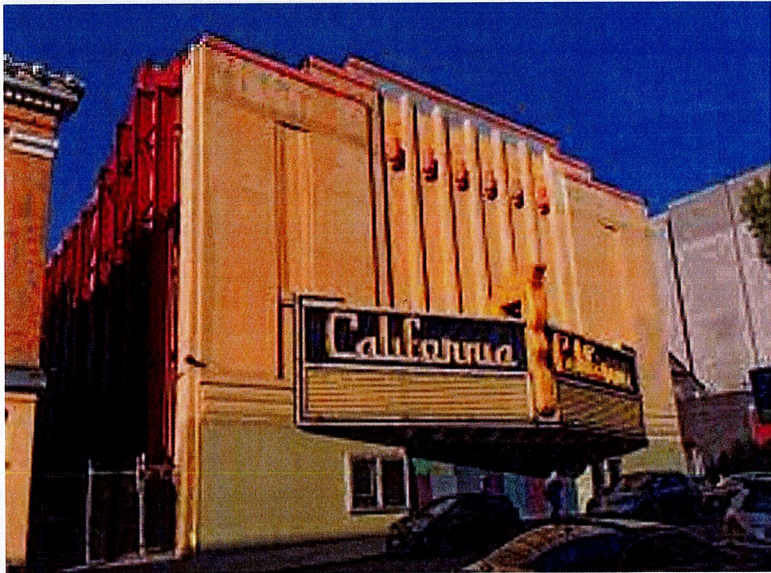
EXISTING THEATER FACADE
