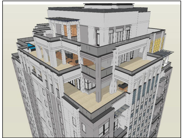
Figure 4: Aerial View of rooftop decks
