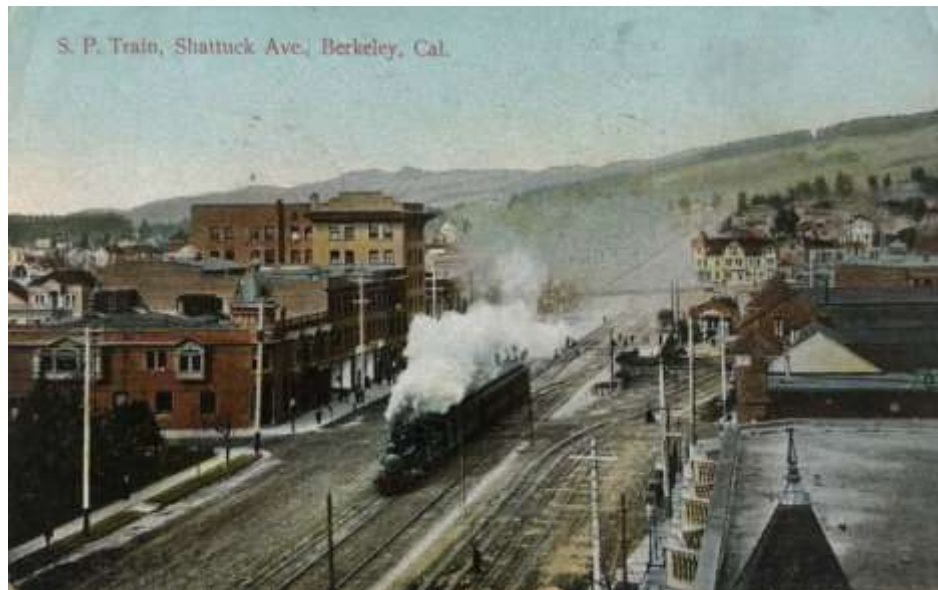
Figure 9. Southern Pacific station on Shattuck Avenue, circa 1909
