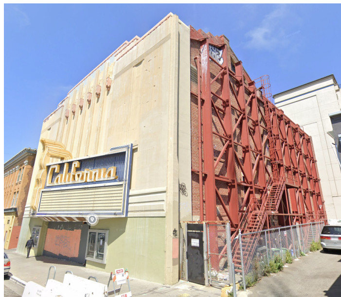
Figure 1: Existing East Facade (URM with Steel Frame)
