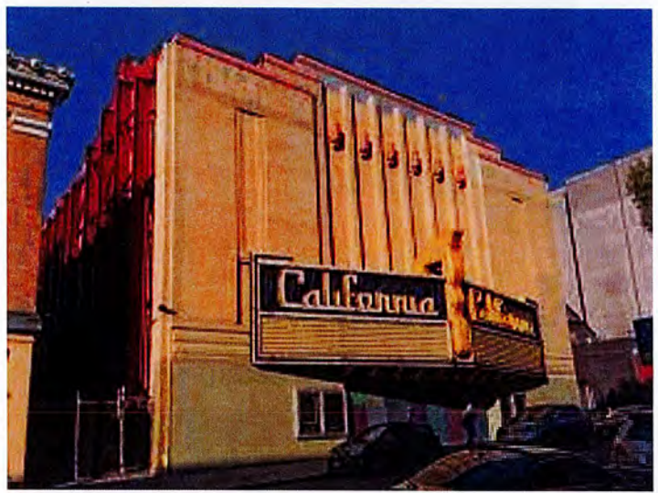
EXISTING THEATER FACADE
