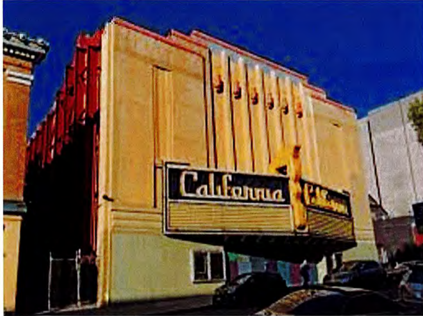
EXISTING THEATER FACADE
