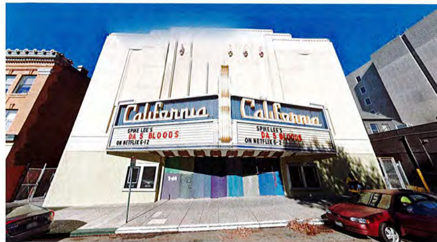
4 STREET VIEW LOOKING NORTHWEST
