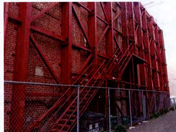
5 EAST SIDEYARD LOOKING WEST
