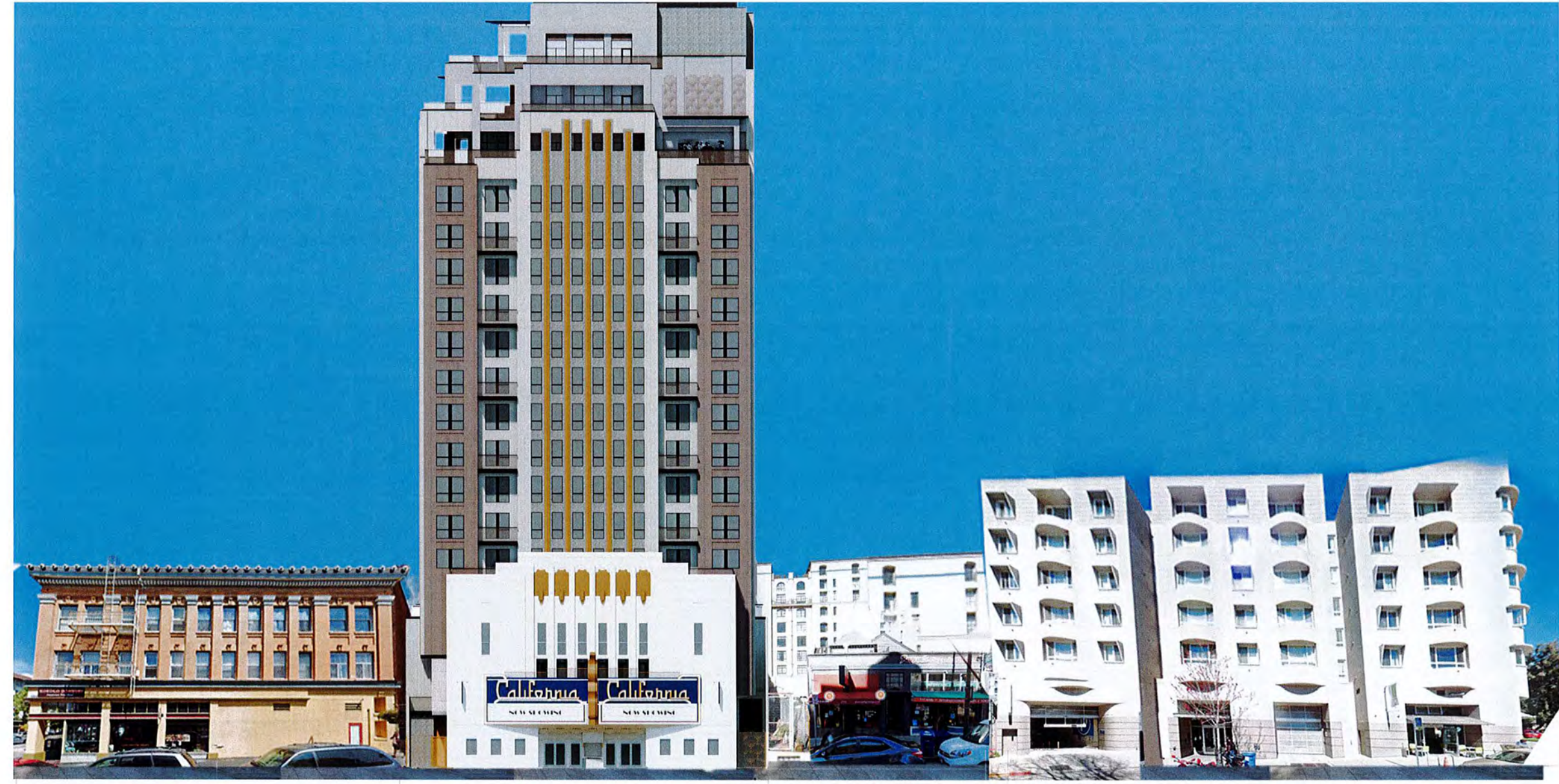
2231 SHATTUCK 2115 KITGREGGE BUILDING SITE 2119 KITTREDGE 2165 & 2177 KITTREDGE
