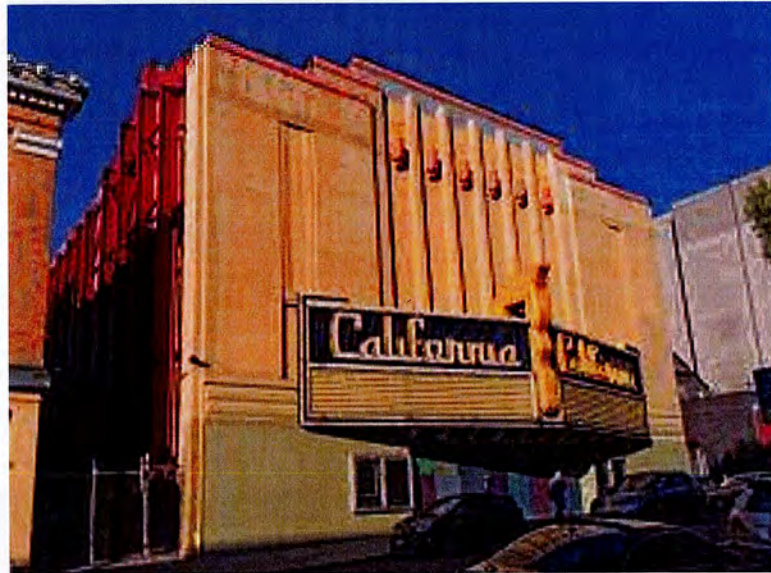
EXISTING THEATER FACADE
