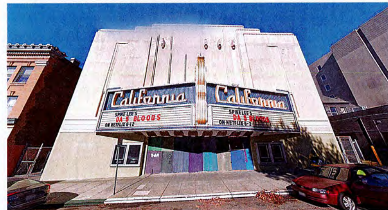
4 STREET VIEW LOOKING NORTHWEST
