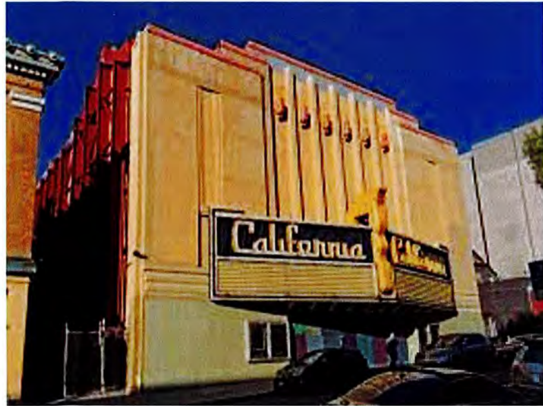
EXISTING THEATER FACADE
