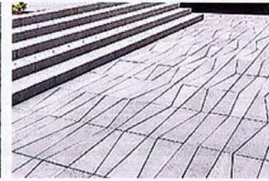
COLORED CONCRETE WITH DECORATIVE SCORING AND SILICA CARBIDE
