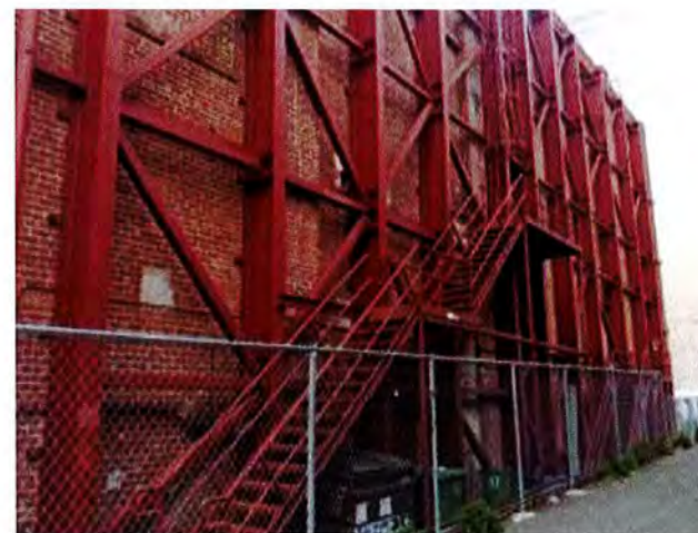
5 EAST SIDEYARD LOOKING WEST
