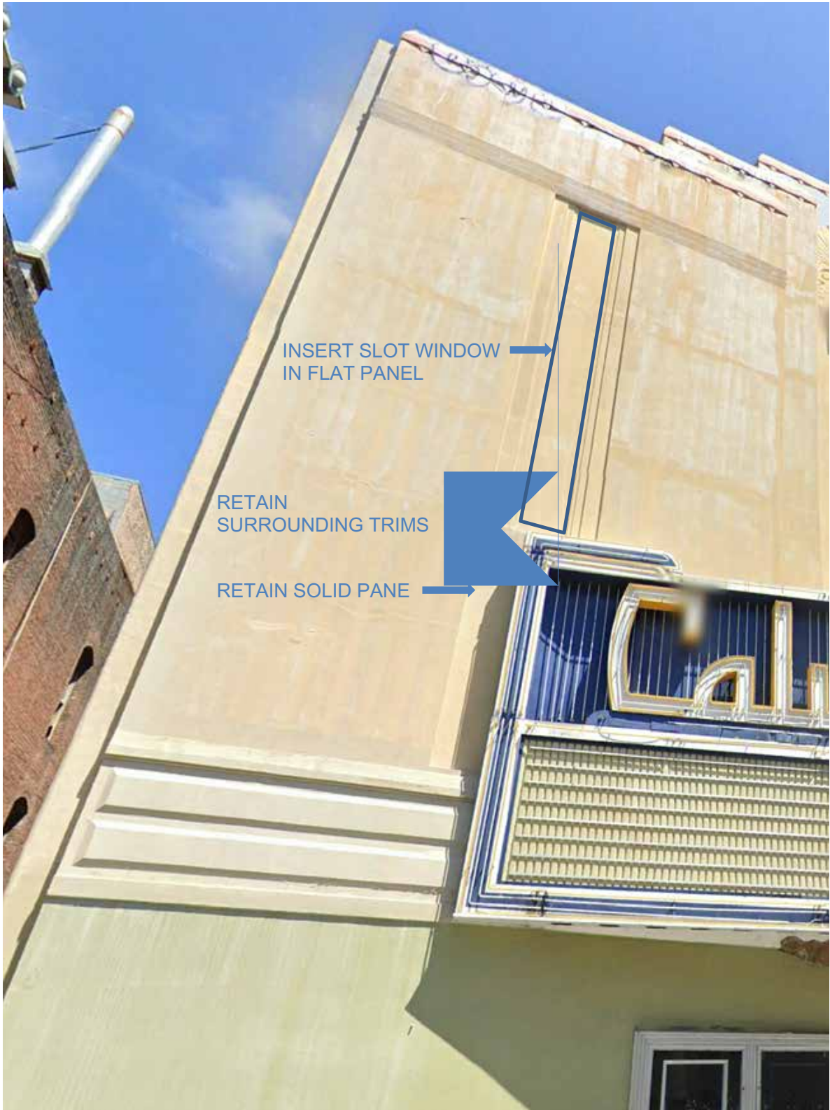
Fig.6 – California Theatre – Recommended window treatment
