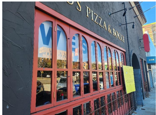
Figure 3: Oblique view of east façade. Looking northwest.
