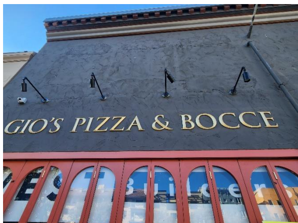
Figure 6: Detail of former tenant signage, lighting, and cornice. Looking west.
