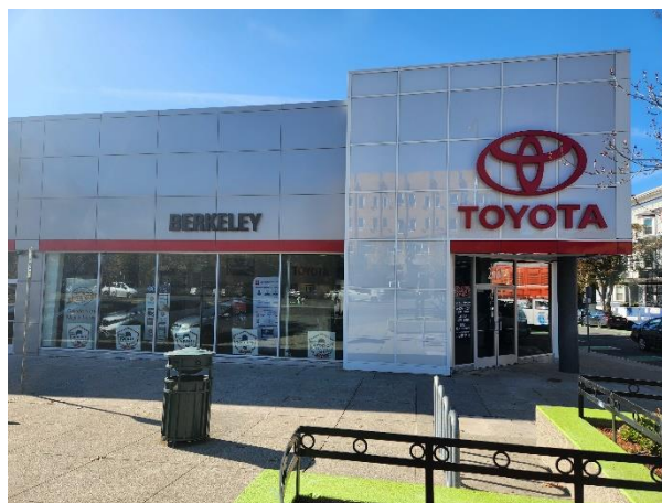
Figure 11: One-story auto dealership at north of subject parcel on Shattuck Avenue. Looking west.
