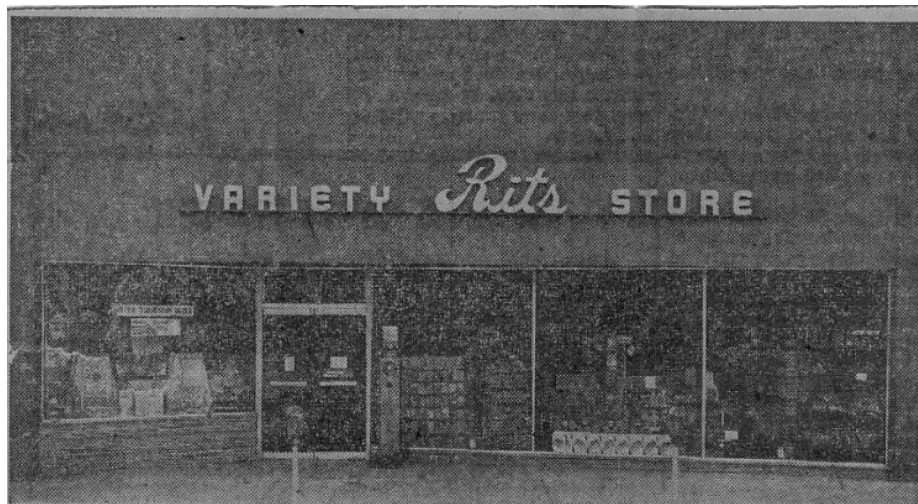
Figure 20. Historic photograph from circa 1952, showing earliest known condition of the primary façade. Note that the storefront windows, bulkheads, and doors are all non-original in this photo. Source: Berkeley Architectural Heritage Association.
