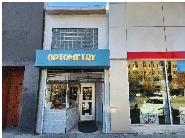
Figure 10: Adjacent one-story optometrist office at 2414 Shattuck Avenue, built 1948. Looking west.
