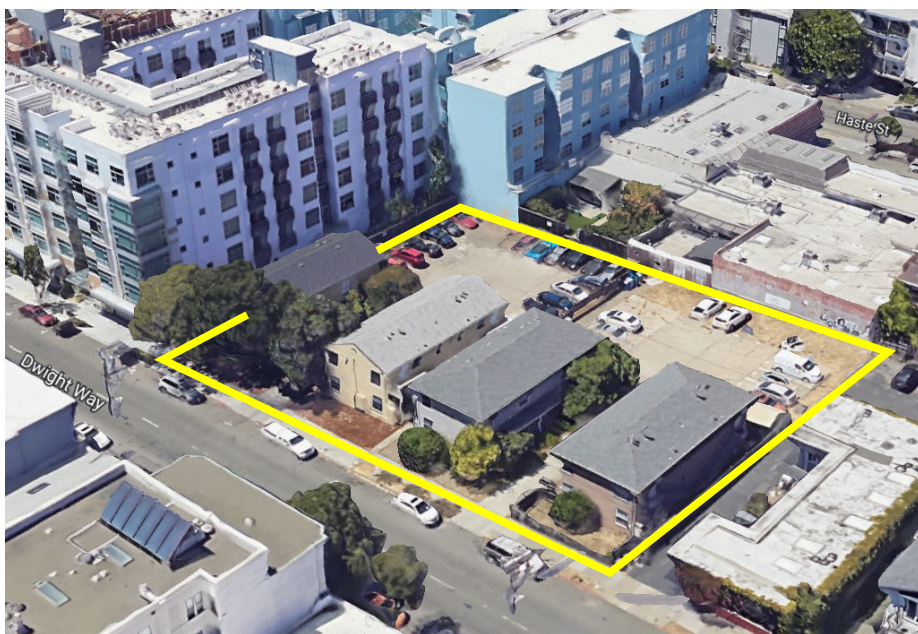
Figure 4. View of the Existing Site
