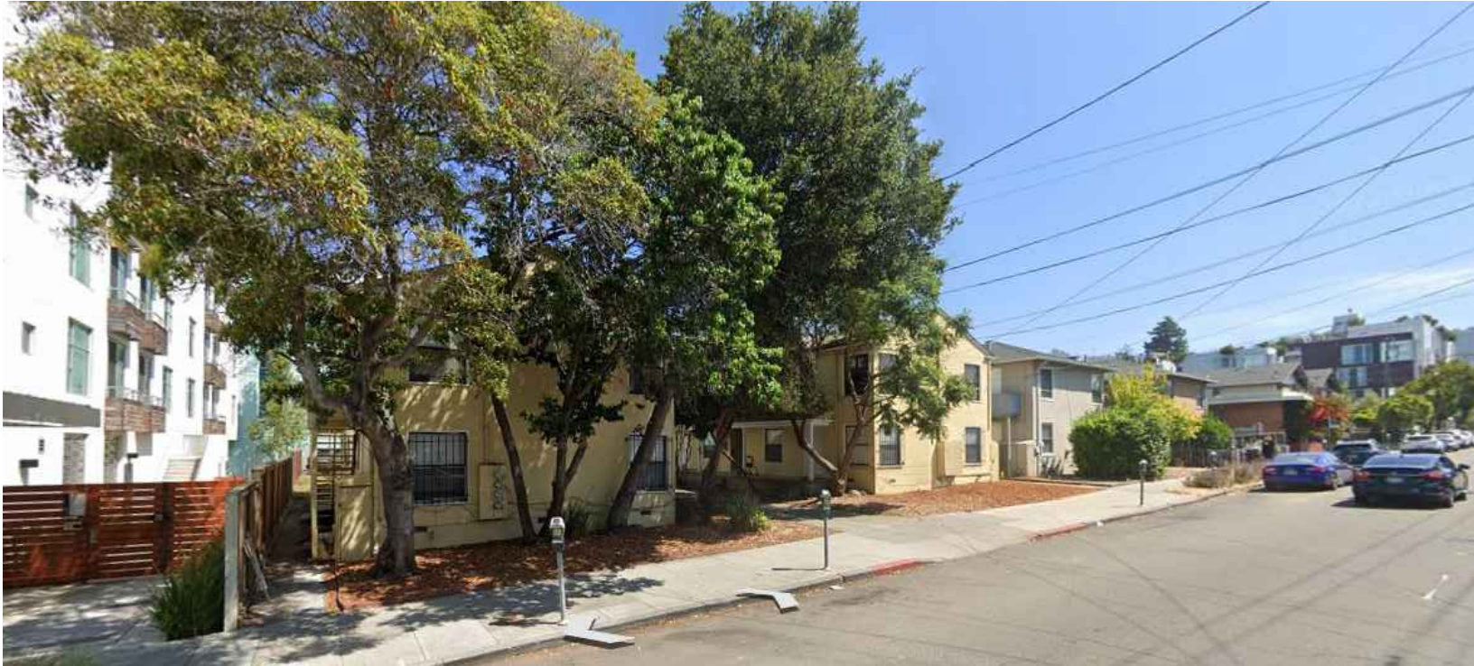
3. SITE (LOOKING NORTH-EAST FROM DWIGHT WAY)
