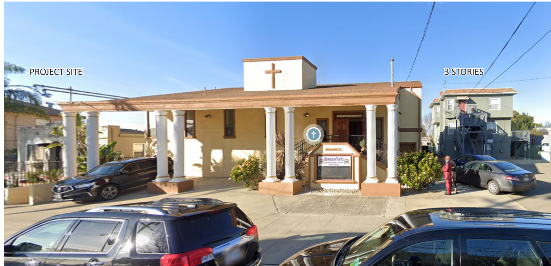
3-STORY MULTI-FAMILY STRUCTURE (2) LOTS AWAY
