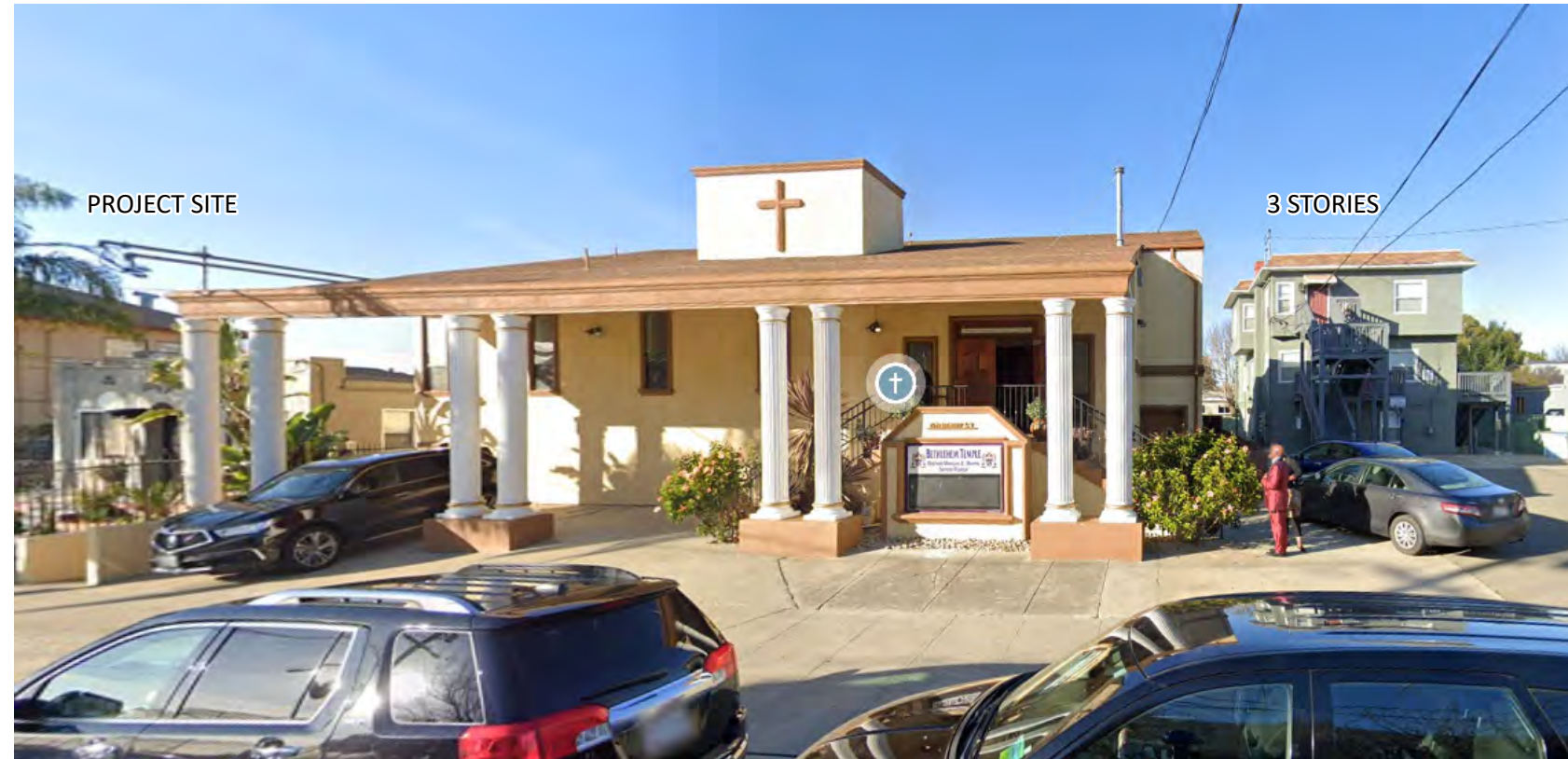
3-STORY MULTI-FAMILY STRUCTURE (2) LOTS AWAY
