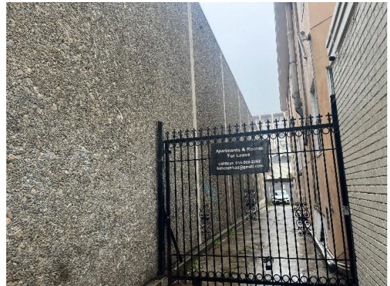
Figure 13: View of west facade, looking south.
