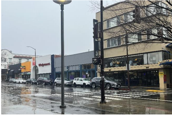
Figure 14: 2470, 2480, and 2486 Bancroft Way, east of subject building.
