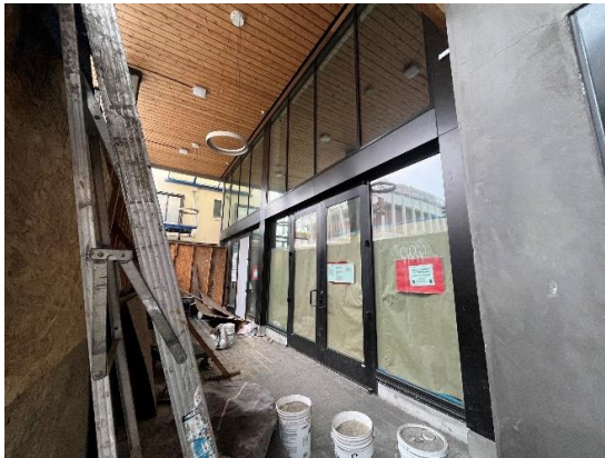
Figure 2: Oblique view of north facade, looking west.
