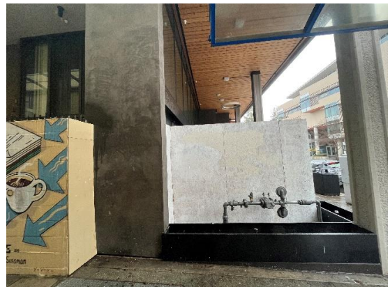
Figure 9: View of north end of east facade, looking west.
