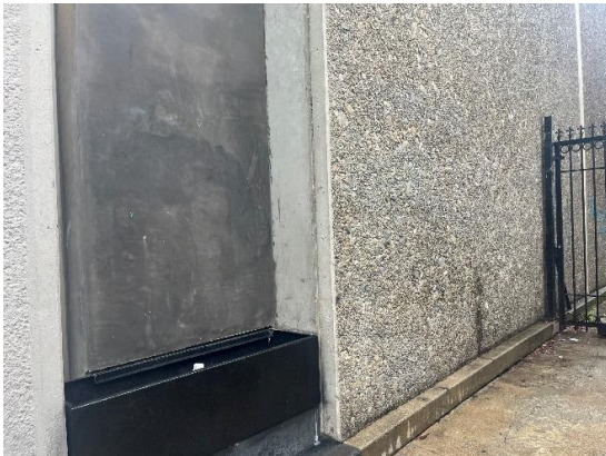
Figure 12: View of north half of west façade, looking south.
