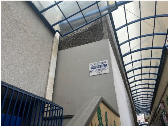
Figure 10: Oblique view of southeast corner of south facade, looking north.
