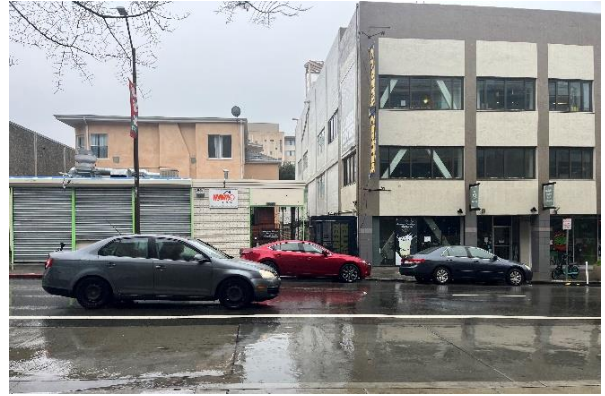
Figure 15: 2456 and 2436 Bancroft Way, west of the subject building.
