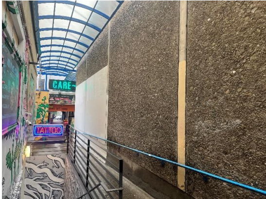
Figure 6: View of east facade, looking south.
