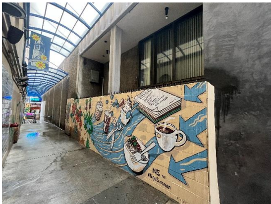
Figure 8: View of east facade, looking south.
