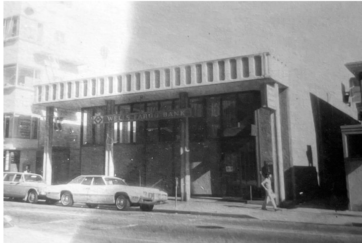
Figure 20: Photograph of 2462 Bancroft Way, 1970s. Source: Berkeley Architectural Heritage Association.
