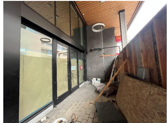
Figure 3: Oblique view of north facade, looking east.
