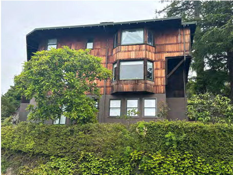
SUBJECT PROPERTY : WEST FRONT FACADE
