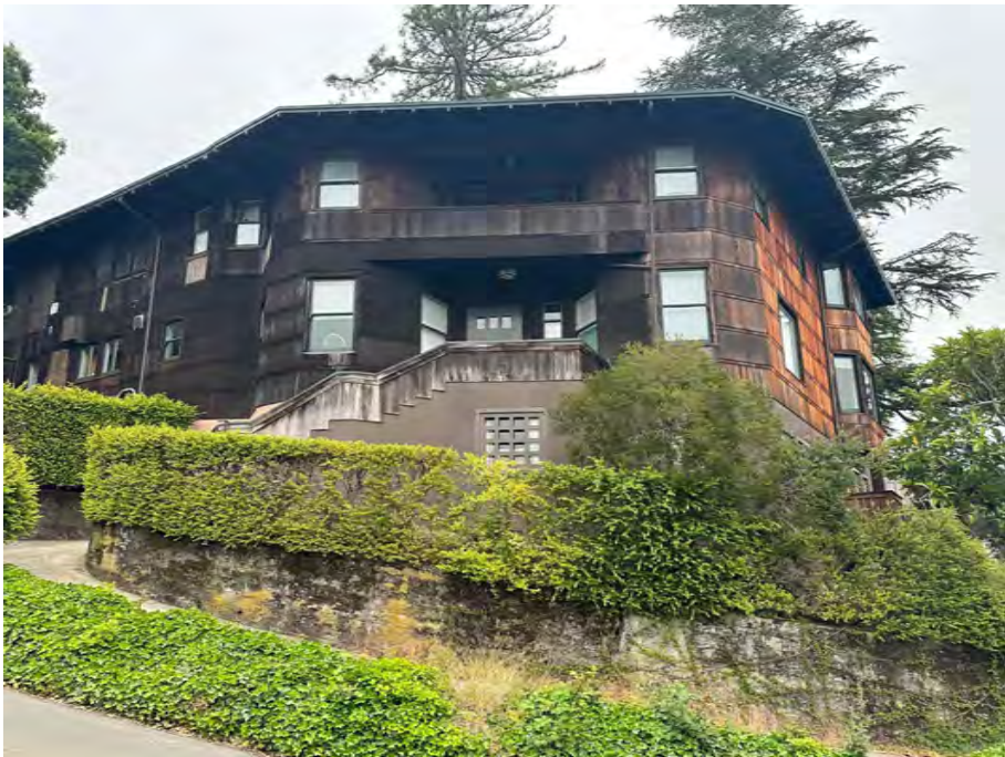
SUBJECT PROPERTY : NORTH WEST CORNER FACADE
