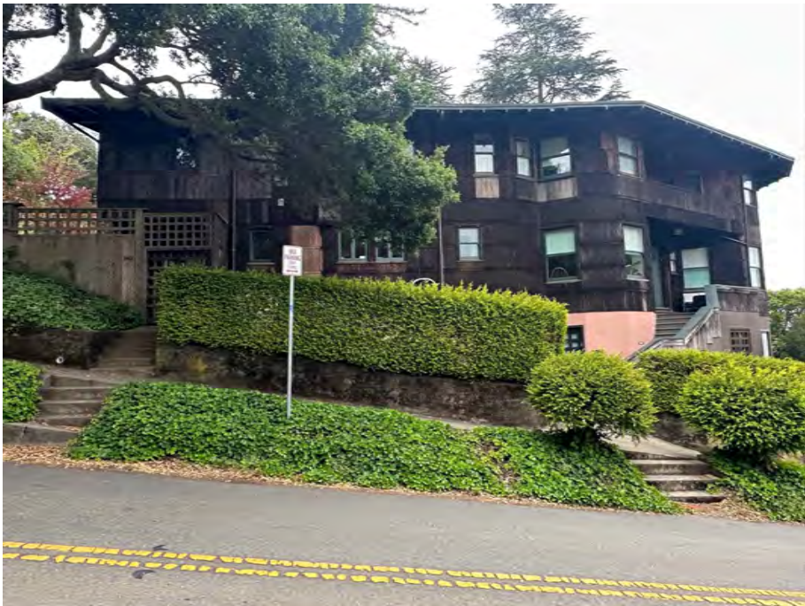
SUBJECT PROPERTY : NORTH FRONT FACADE
