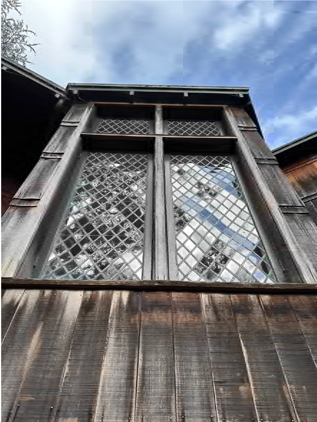
Windows at JGH stair.
