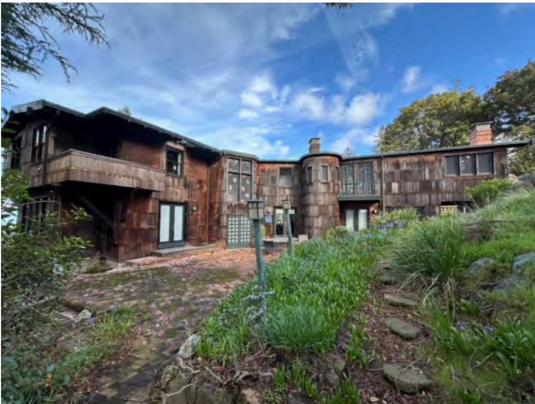
Garden view of the south end and stair tower
