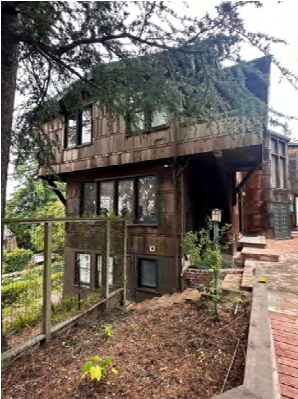
Courtyard view of the south end elevation with leaded glass windows
