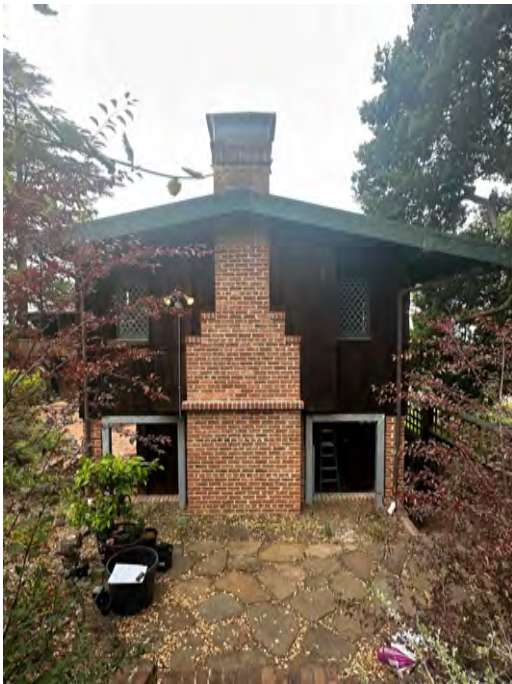
SUBJECT PROPERTY : EAST SIDE FACADE
