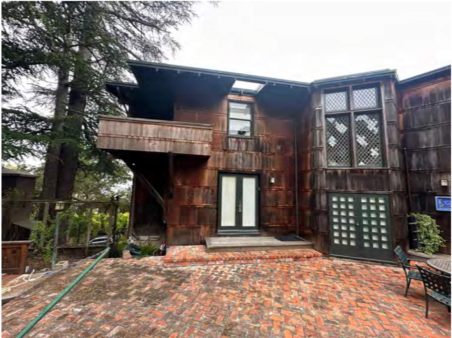
SUBJECT PROPERTY : EAST INTERIOR FACADE
