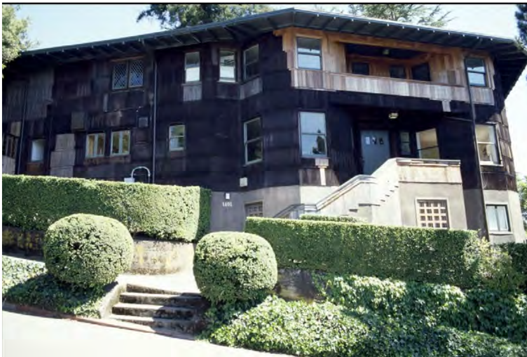
View of main entrance at corner of Le Roy Avenue & Rose Street (2001) (note: replacement shakes in cedar.)
