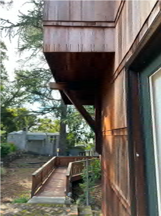
Note: Wood braces on south balcony as model to brace the JM balcony.
