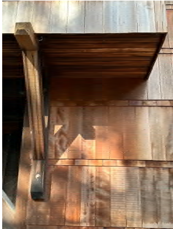
Note: Wood braces on south balcony as model to brace the JM balcony.
