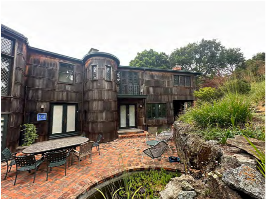
SUBJECT PROPERTY :SOUTH INTERIOR FACADE
