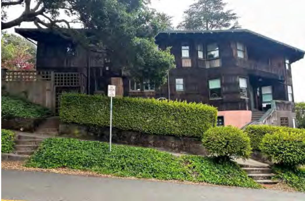
Figure 4: Current site conditions – Front (north) elevation (Denise Hall Montgomery Architecture, 2024)
