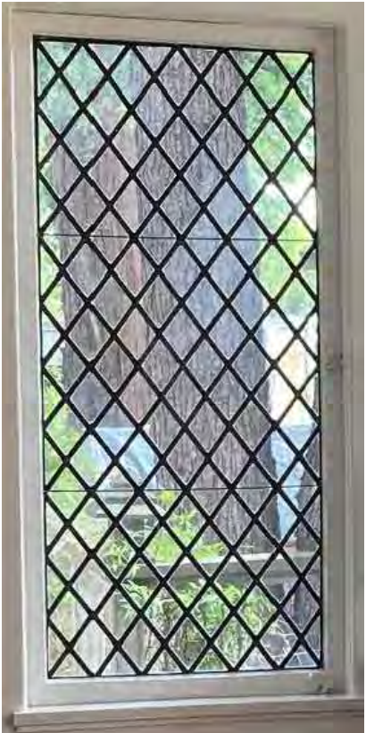
INTERIOR FINISHES: LEADED GLASS WINDOW RESTORATION TO MATCH EXISTING WHITE SASH AND FRAME
