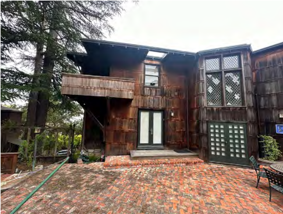
Courtyard view of the south end and stair tower
