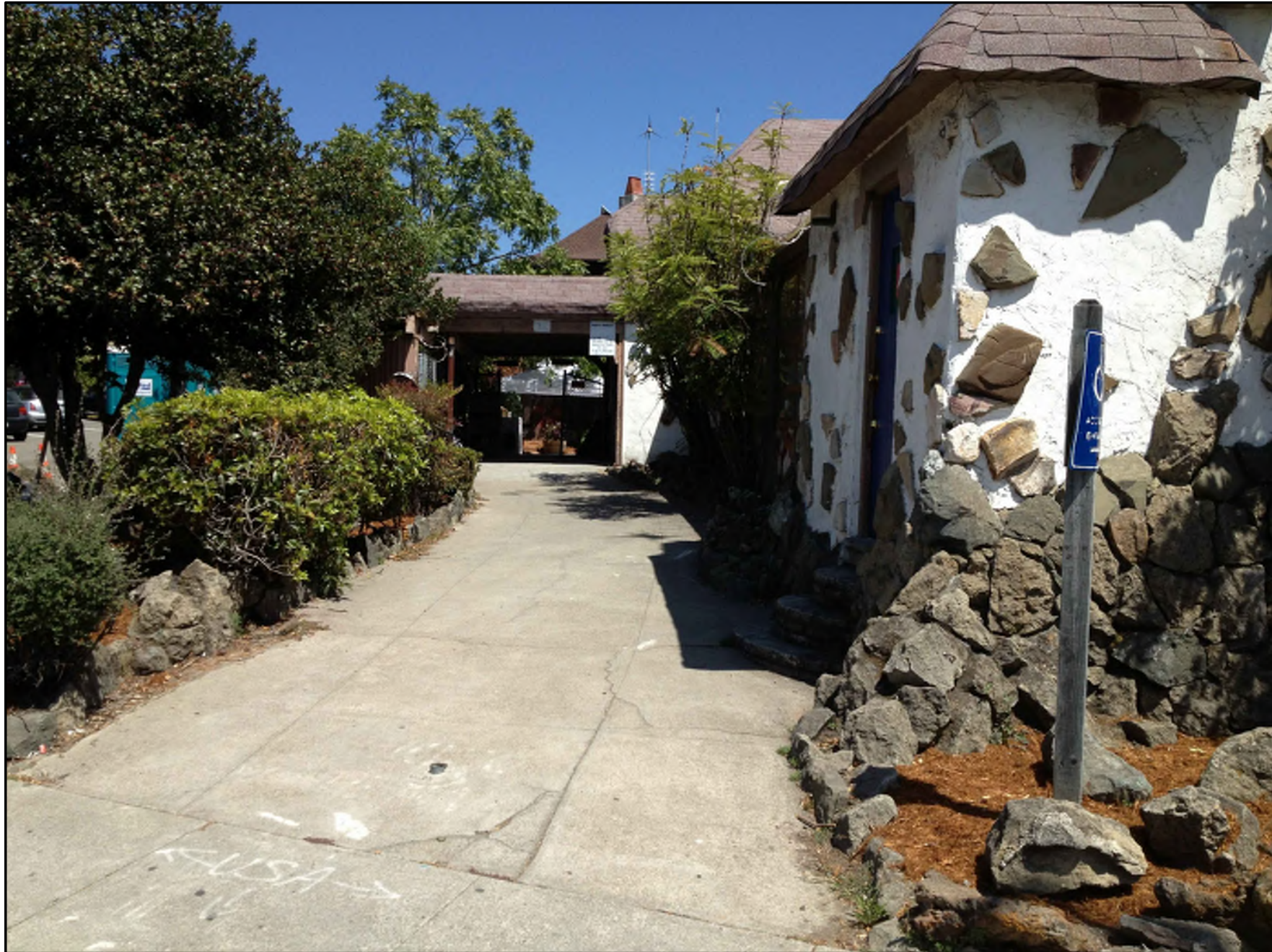
Adjacent Existing driveway @3049 Adeline street
