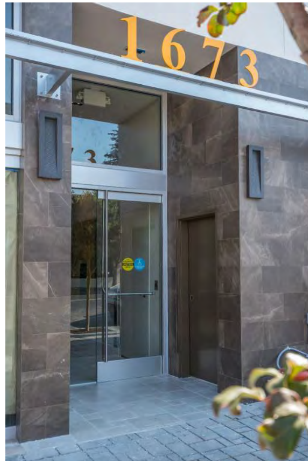
EXTERIOR COLOR AT METAL CANOPY & COLUMN AT FRONT ENTRY
