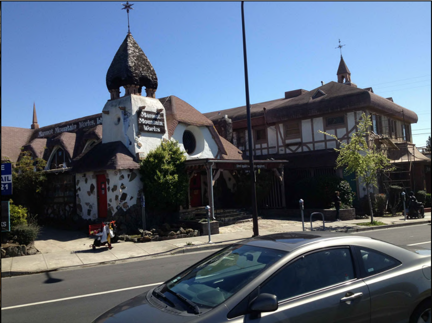
3049-3051 Adeline street- existing Buildings
