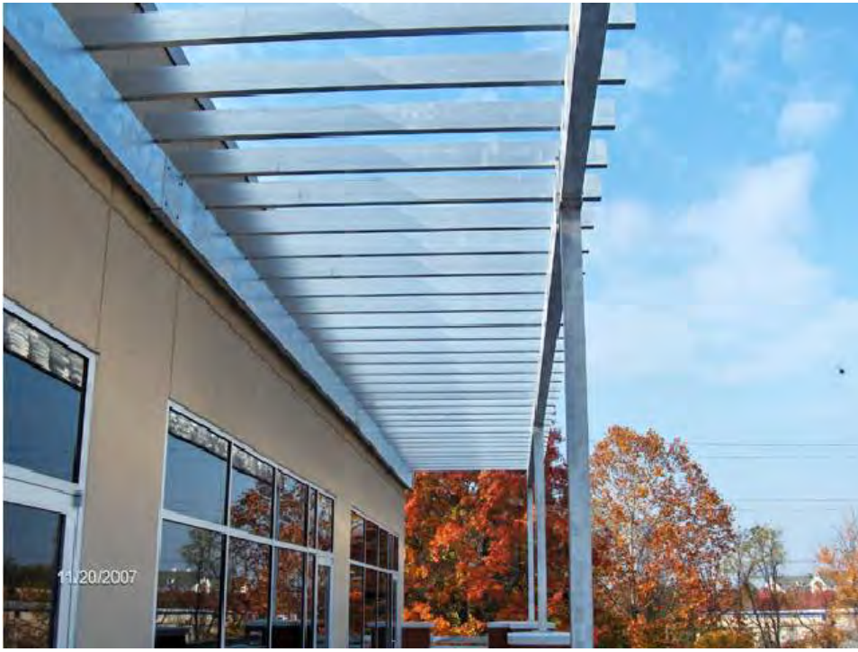
ALUMINIUM TRELLIS AT TOP FLOOR
