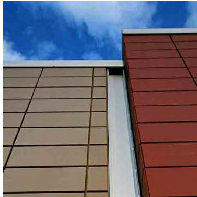
EXTERIOR PANEL CLADDING by shildan or eq.
