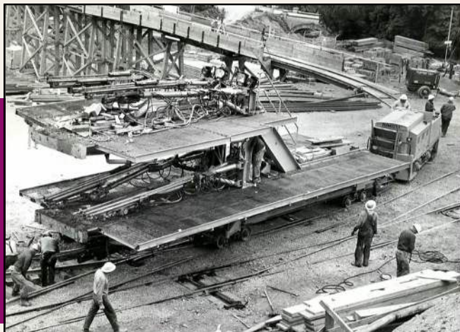
"Jumbo" tunnel digger for construction of Berkeley BART line
