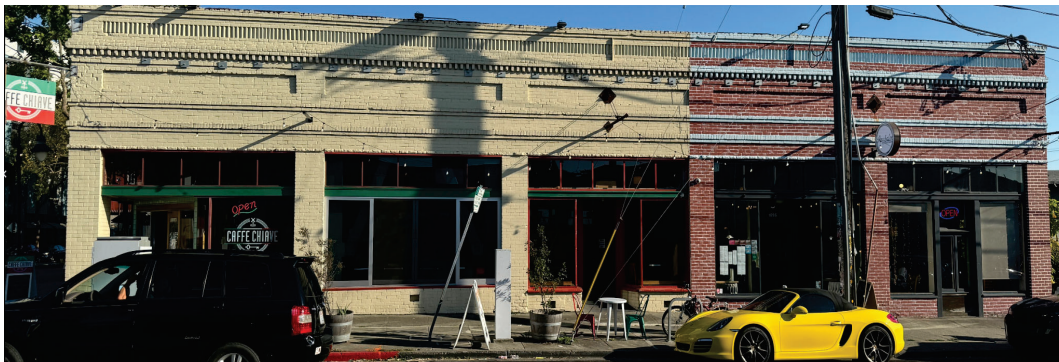
Photo showing the series of storefronts along the north elevation facing south
