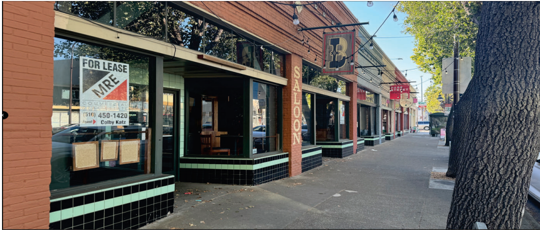
Photo showing the series of storefronts along the east elevation facing north
