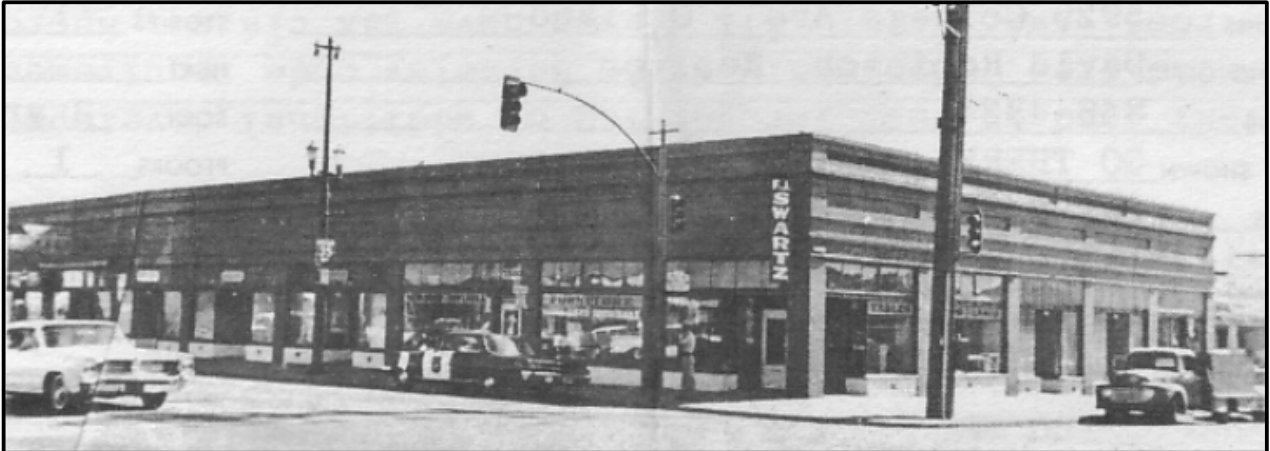
Figure 2: Subject Building – Site Conditions circa 1960 (Berkeley Architectural Heritage Association)
