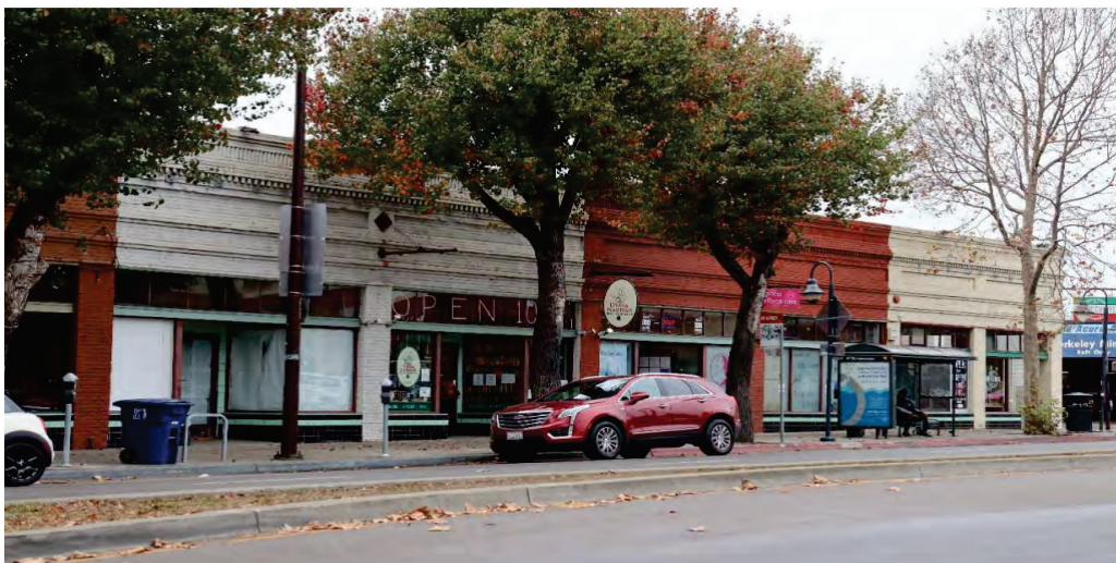
East elevation (primary facade) of the 1907 storefront commercial building, facing northwest.
