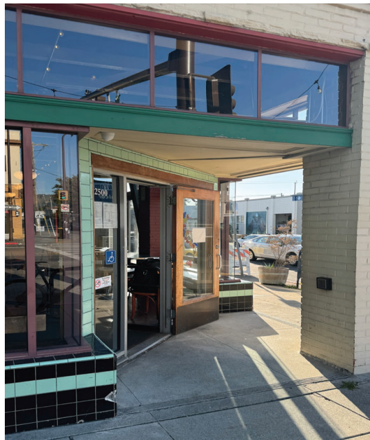
Entryway at corner of San Pablo and Dwight Way
