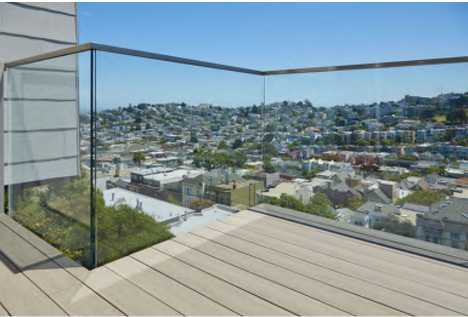
GLASS GUARDRAIL SYSTEM
