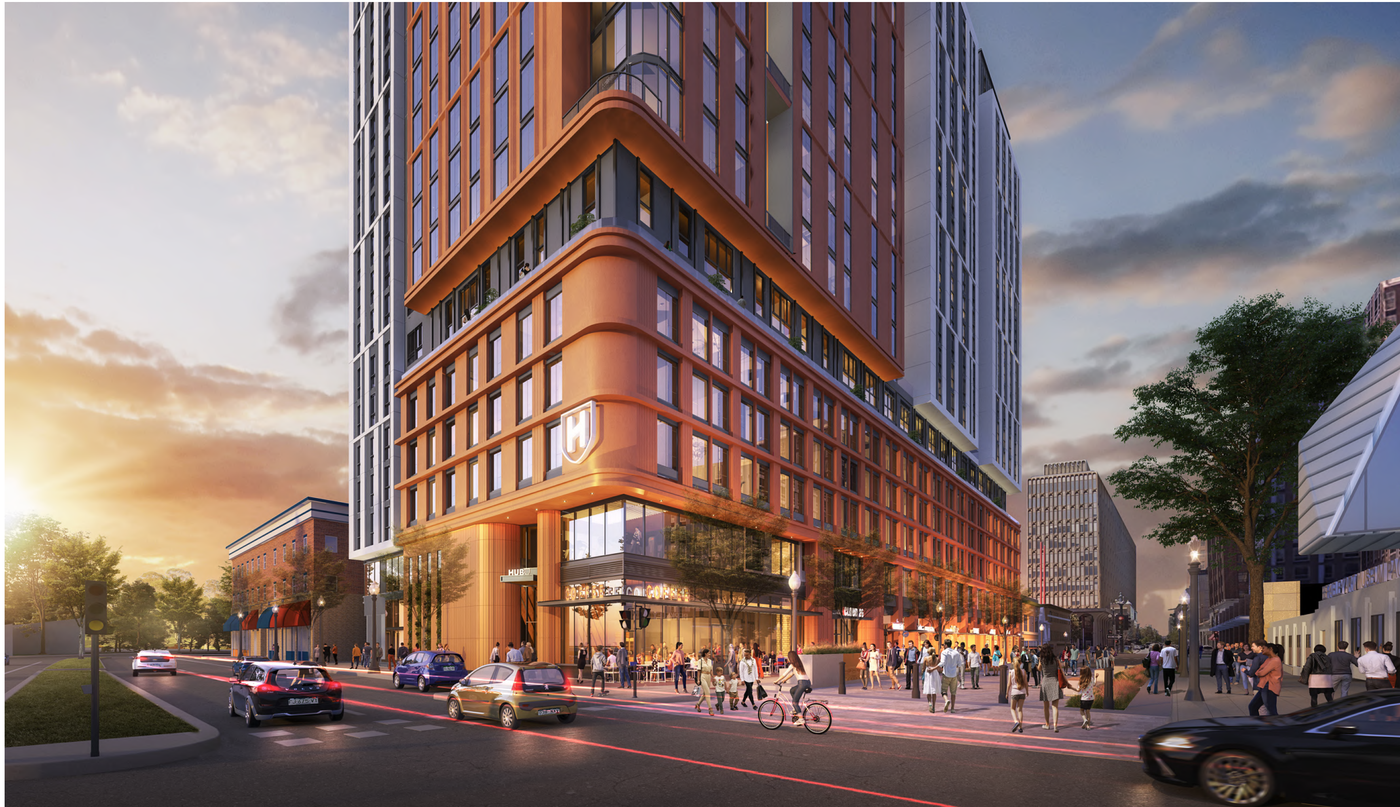
CORNER VIEW FROM OXFORD ST & CENTER ST
