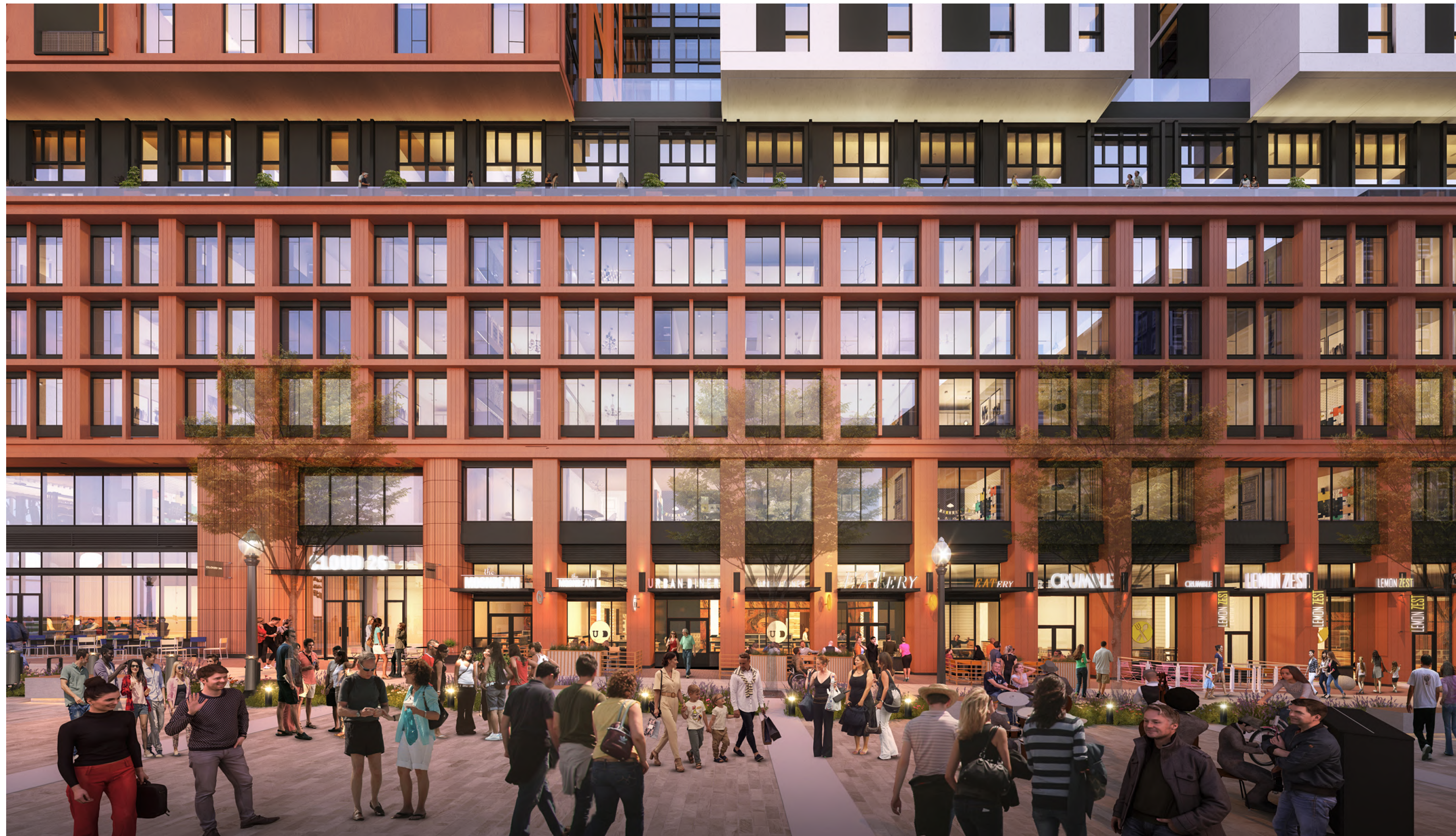
CLOSE-UP OF FACADE ON CENTER ST.
