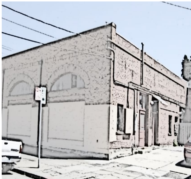
Exhibit 7. Example of unreinforced masonry construction
