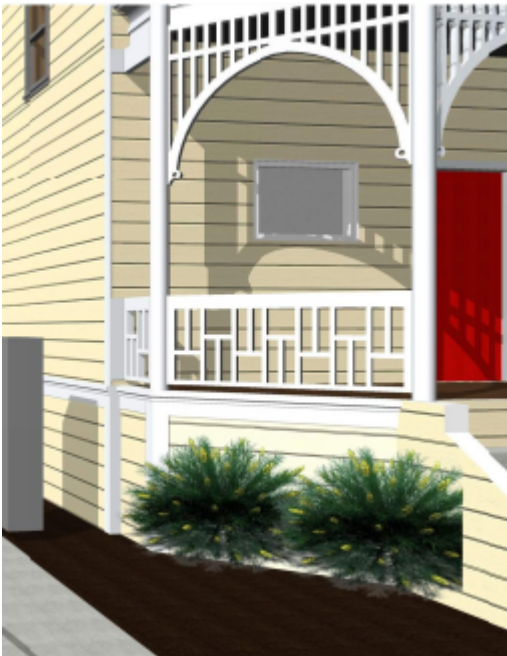
Figure 10: restored wood filigree arches at porch
