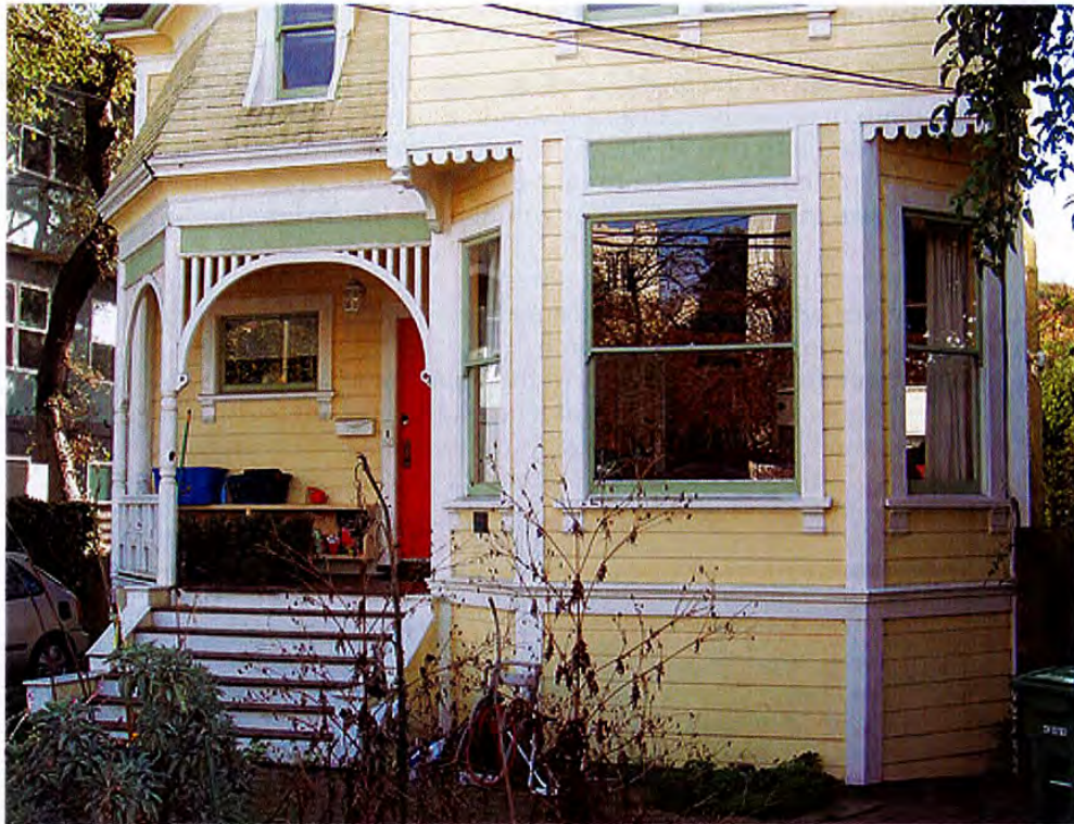
Figure 15. Ground floor, front façade
