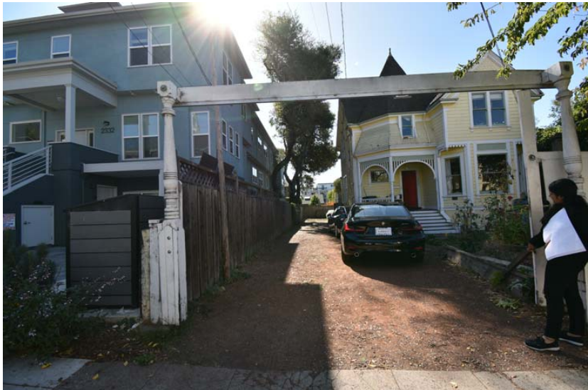
E - EXISTING DRIVEWAY AND ADJACENT BUILDING
