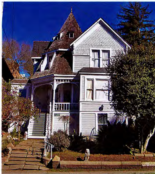
Figure 55. J.L. Donovan House (c. 1898), 1431 Arch Street
