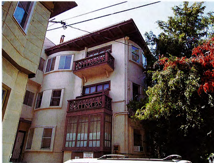
Figure 104. Balconies at 2410 Dana Street, 2007
