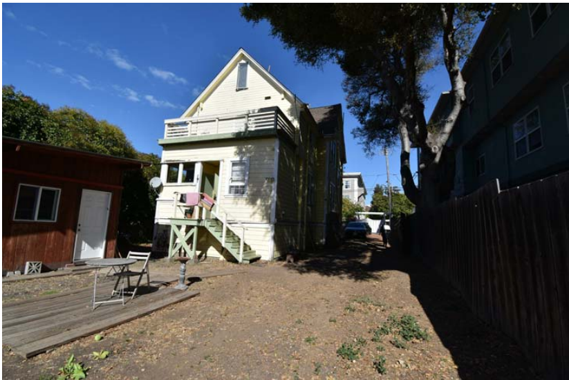
C - EXISTING BACK OF HOUSE
