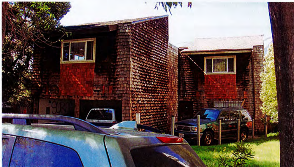
Figure 92. Townhouses at 2402-2404 Dana Street
