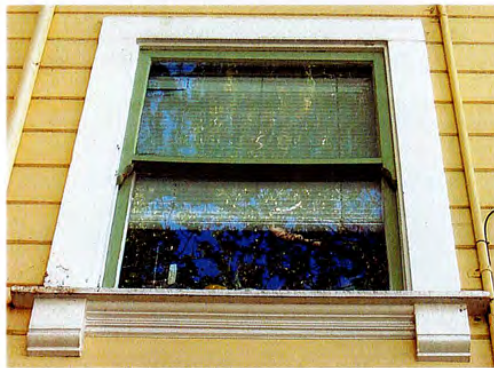
Figure 20. Mid-story window on east façade
