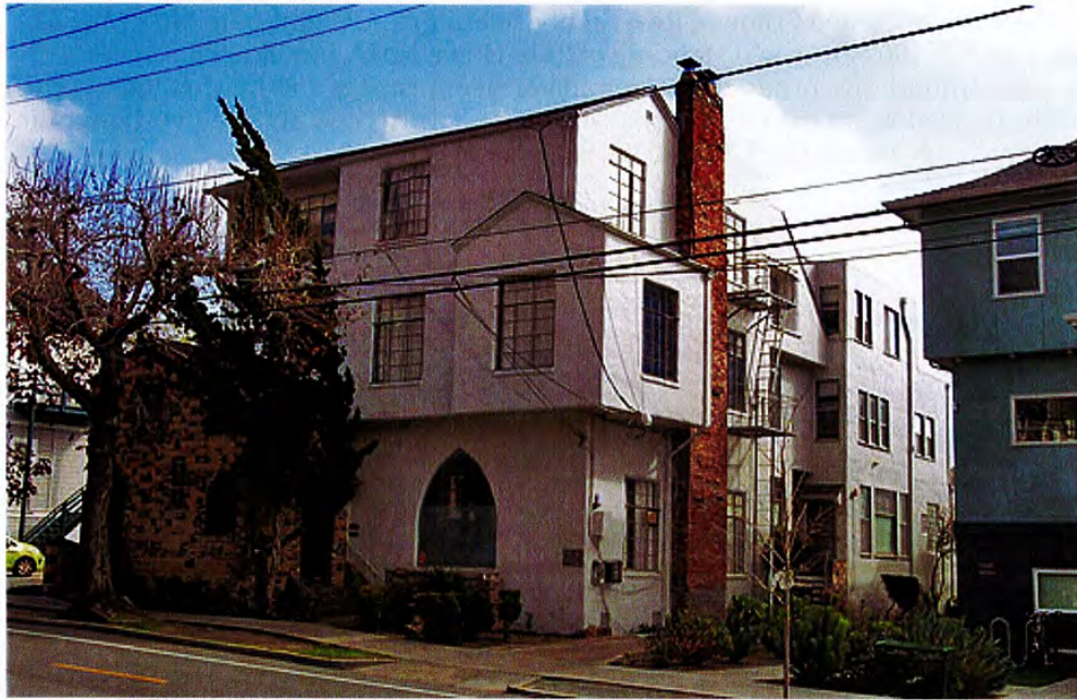
Figure 91. Francis Wood Apartments, 2336-38 Channing Way, in 2020
