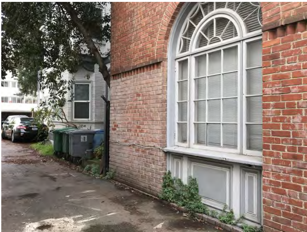
Lower east facade, looking southwest.
