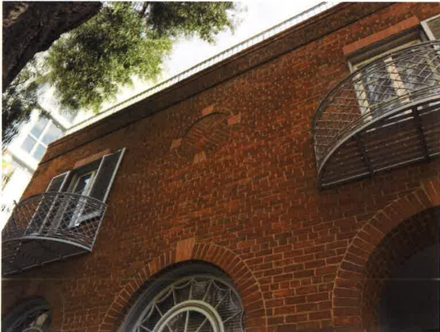
Second story of primary facade.
