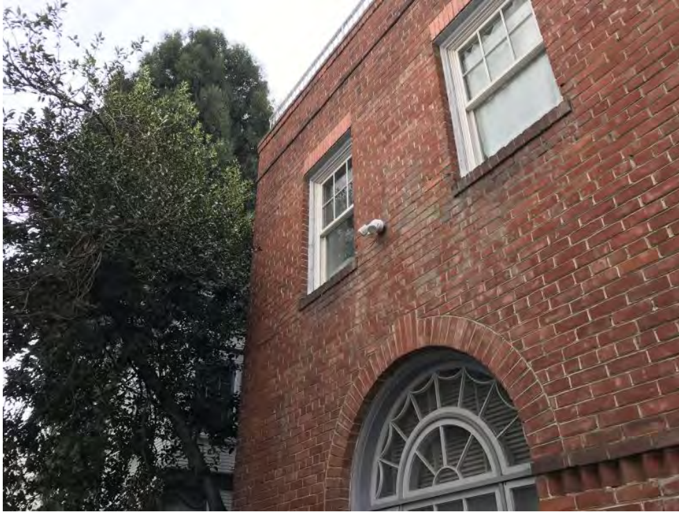
Upper east facade, looking southwest.
