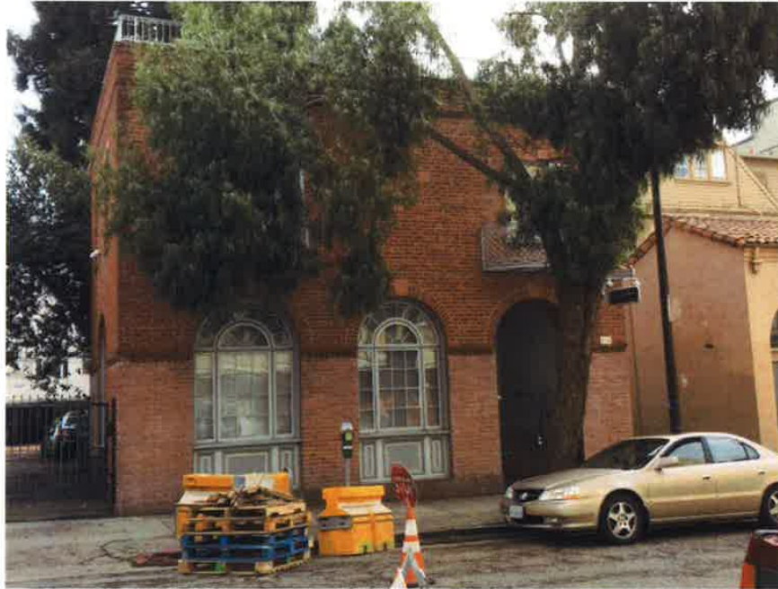
Primary facade, looking south from Kittredge Street.
