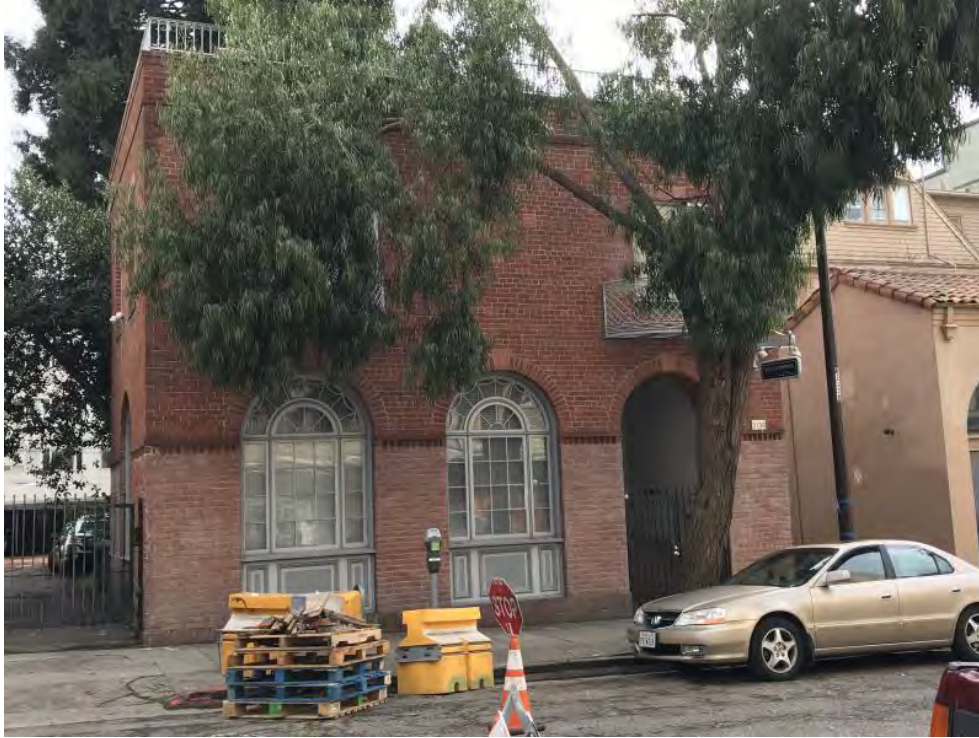
Primary facade, looking south from Kittredge Street.
