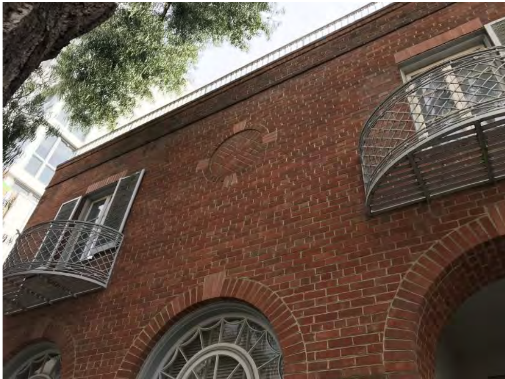
Second story of primary facade.
