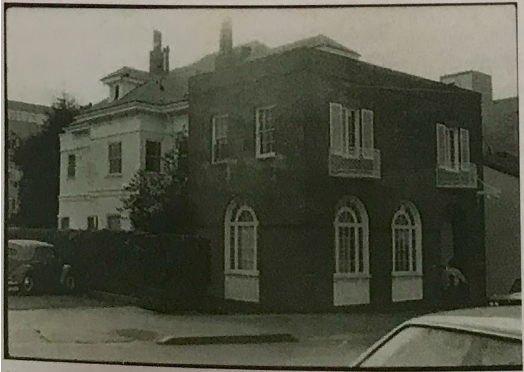
2138 Kittredge Street, looking southwest; 1978. (BAHA)
