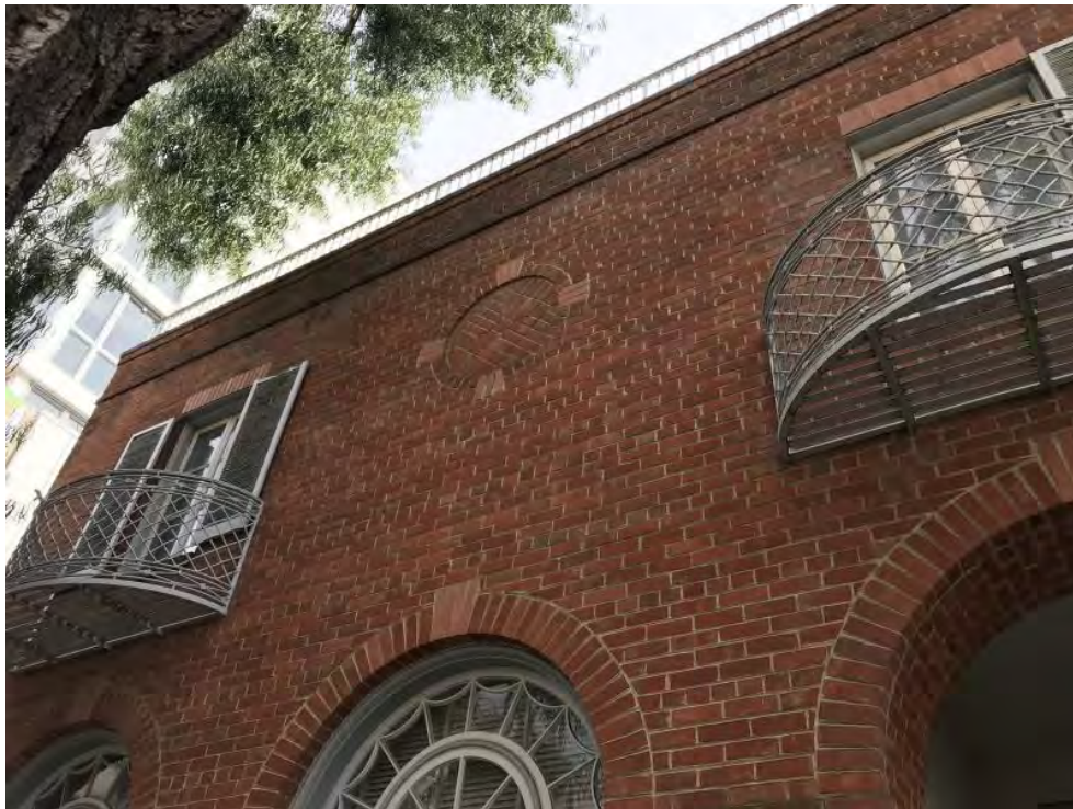
Second story of primary facade.
