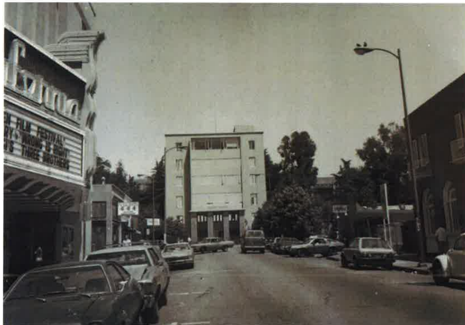
Kittredge Street, looking east. 2138 Kittredge Street at far right; 1982. (BAHA)
