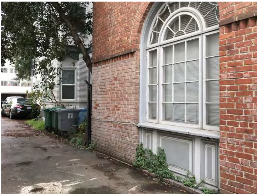
Lower east facade, looking southwest.
