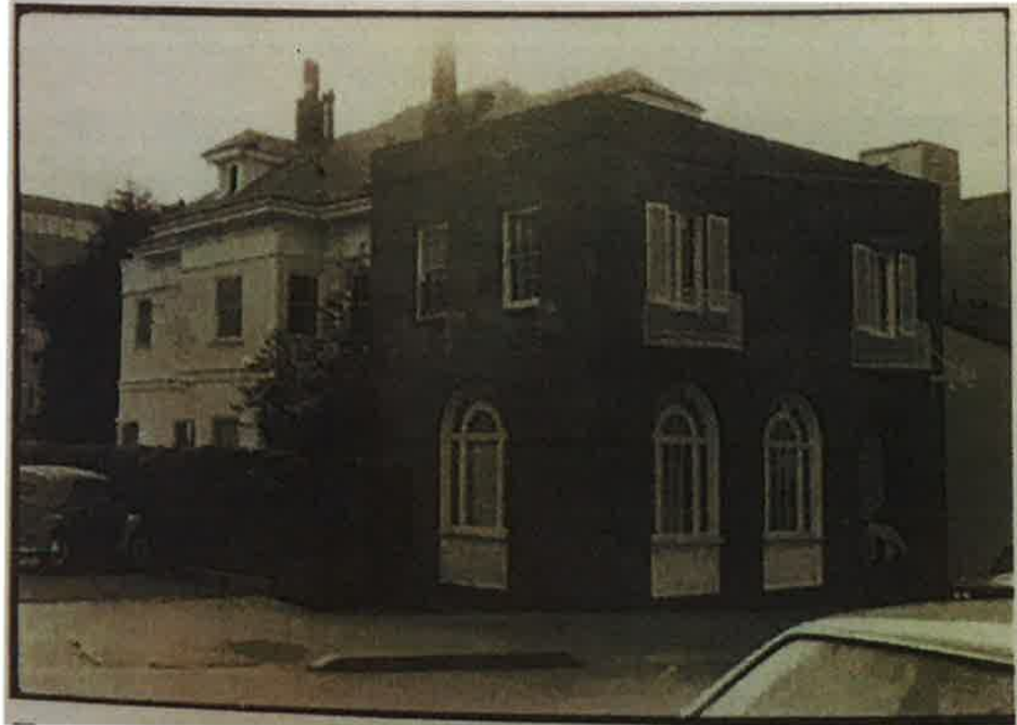
2138 Kittredge Street, looking southwest; 1978. (BAHA)
