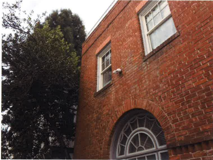
Upper east facade, looking southwest.
