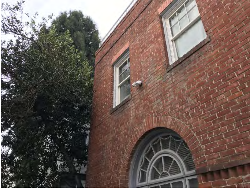
Upper east facade, looking southwest.
