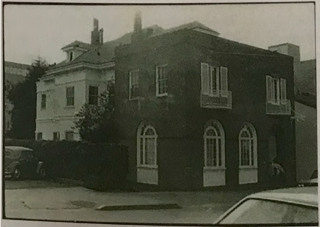
2138 Kittredge Street, looking southwest; 1978. (BAHA)
