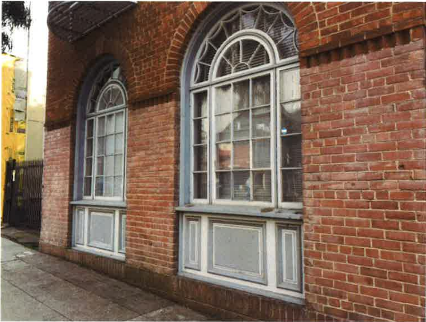
First story of primary facade, left of primary entrance.
