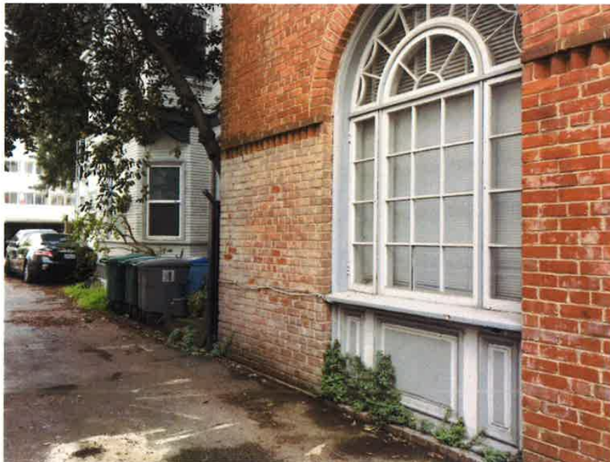
Lower east facade, looking southwest.
