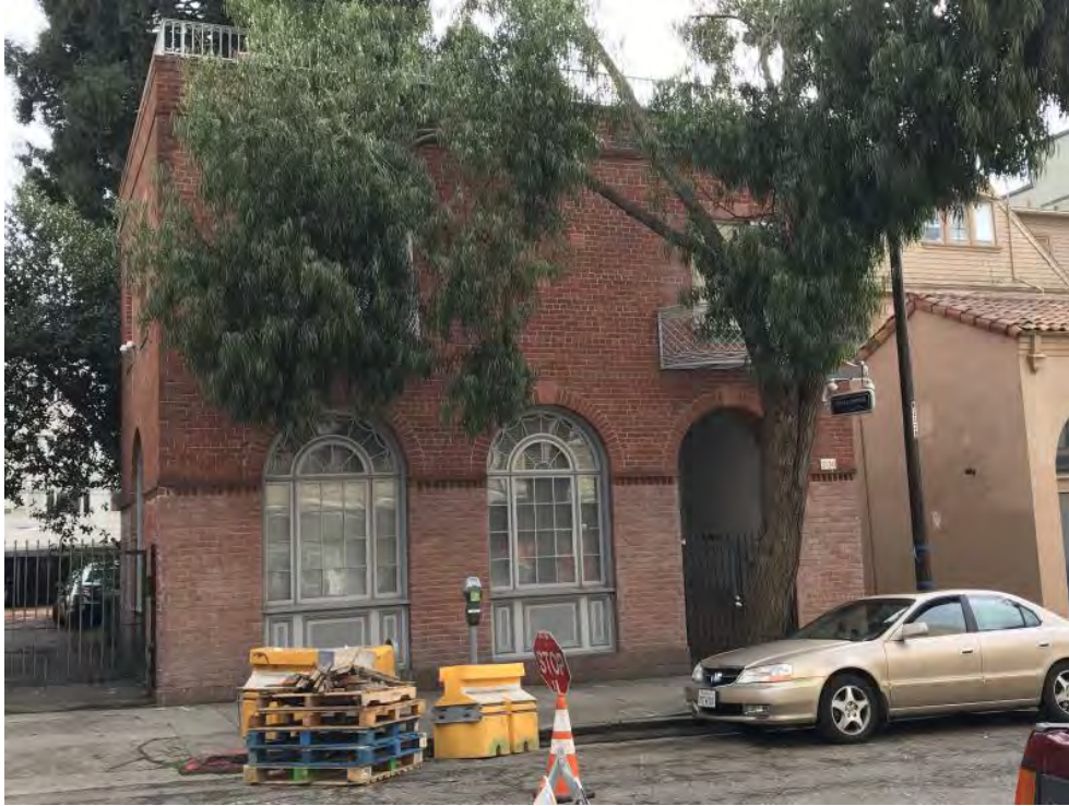
Primary facade, looking south from Kittredge Street.
