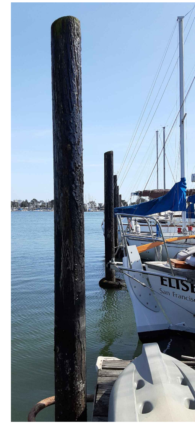
TIMBER PILES PHASE 1 DEMOLITION D-100/D-101
