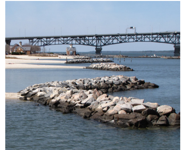
Example of Rock Breakwater | National Park Service
