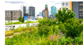
Intensive Green Roof
