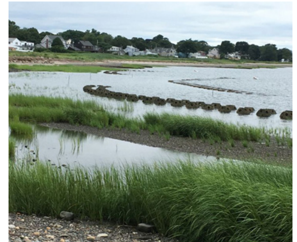
Example of Living Shoreline | Florida Living Shorelines
