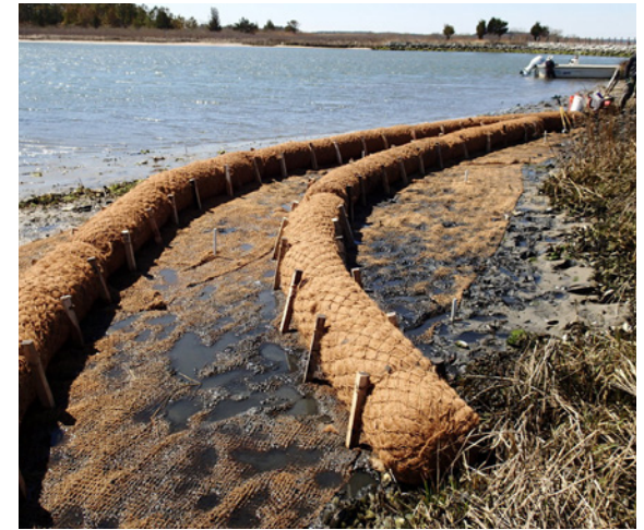
Example of Living Shore Coir Logs | Delaware Living Shorelines
