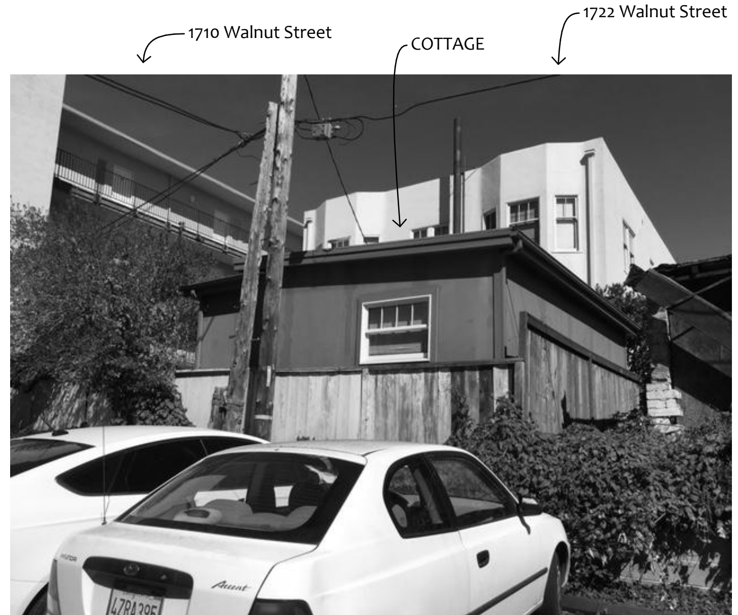
WEST SIDE OF COTTAGE
