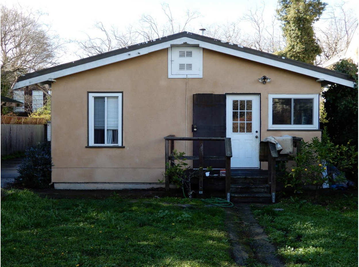
Figure 5. Rear façade, view toward west.
