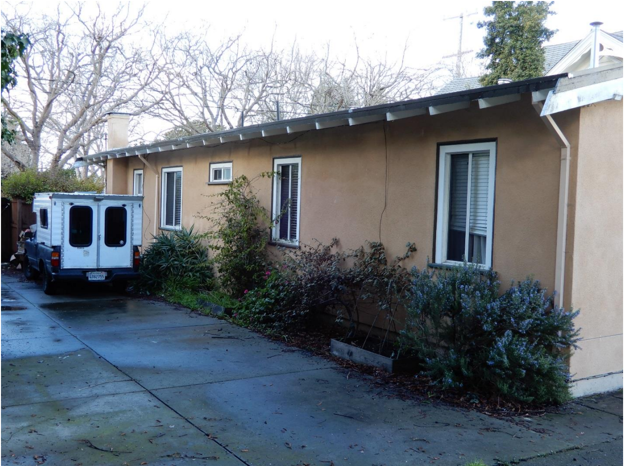
Figure 7. South façade, view toward northwest.
