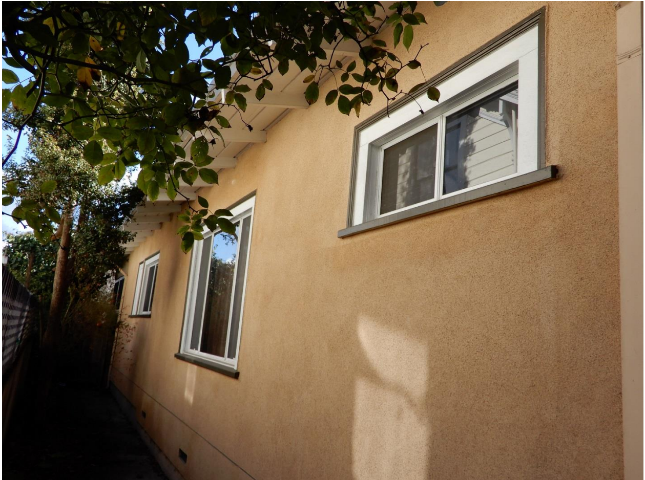
Figure 4. North façade, view facing east.
