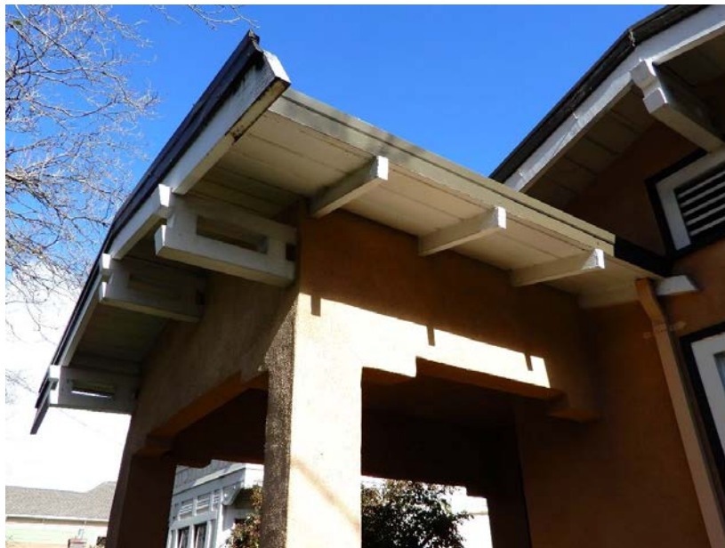
Figure 3. Unenclosed eave overhang at the porch, showing distinctive decorative braces, view facing northeast.
