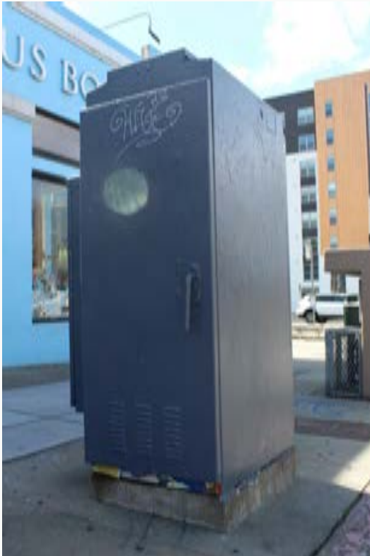
Location: Durant Ave./Shattuck Ave.
