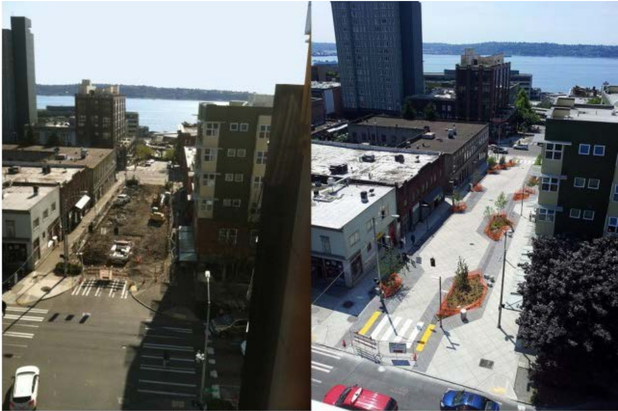
Bell Street, during and shortly after construction.
