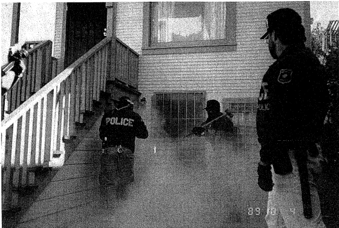
Drug Task Force at work: Officer Gary Romano uses high temperature cutting torch to effect entry to a drug house, while Officers Rosie Brown, with sledge hammer, and Garen Nielsen assist.
