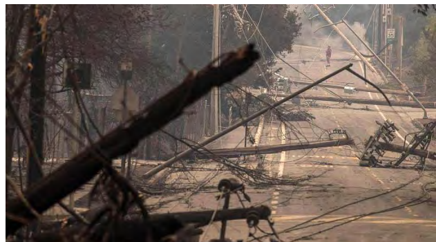
Figure 11 - Downed power poles and lines in 2017 Tubbs Fire Photo by LA Times
