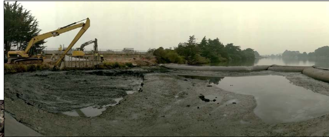
Lagoonside sediment removal and coffer dam
