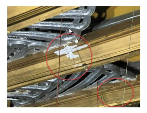
Cracked and spalled plaster in the main auditorium
