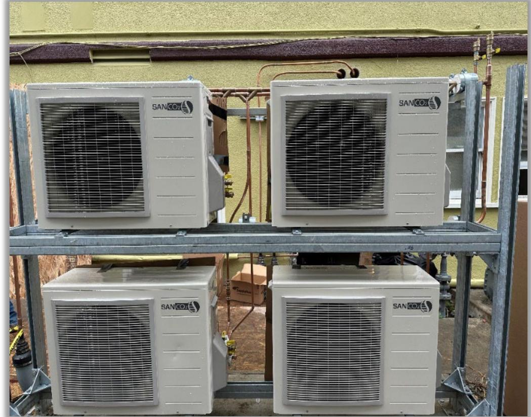
Walnut House Coop heat pumps for the centralized heat pump water heater system, bringing hot water to each of the units
