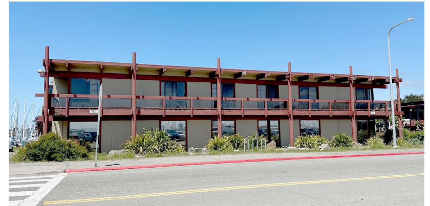
125-127 University Ave. (Office suites & BPD Traffic Bureau)
