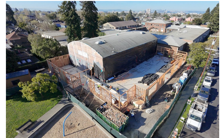
MLK Jr. Youth Services Center (under construction)
