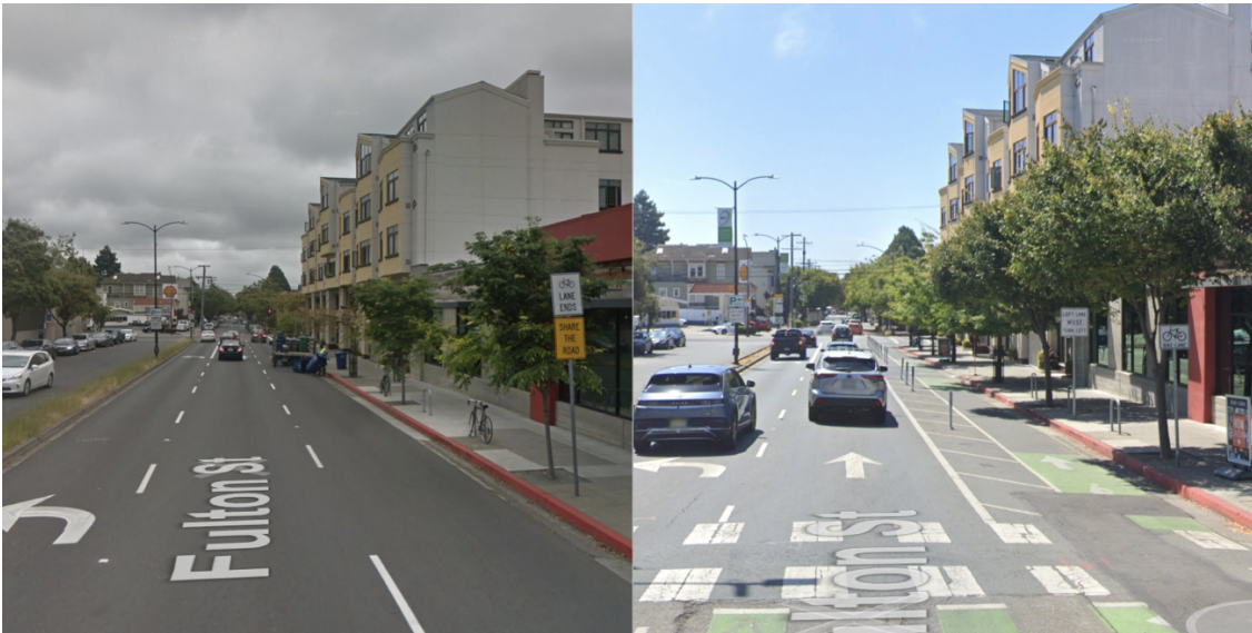
Before-and-after comparison showing the quick-build bicycle facility constructed on Fulton St. in 2016 (Google Street View).
