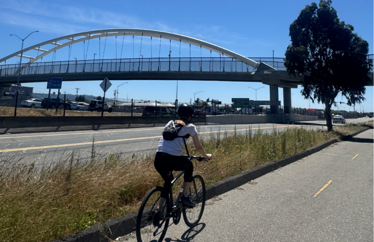
Bridge over I-80 and Gilman Street for people walking and bicycling.
