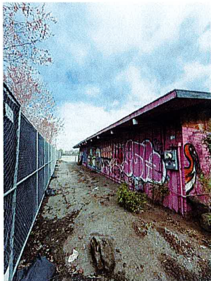
STRUCTURE TO BE DEMOLISHED - WEST ELEVATION
