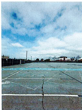
EXISTING PARKING LOT IN SUBJECT PROPERTY
