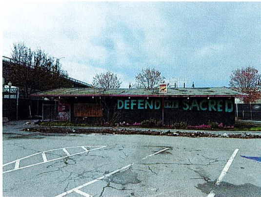
STRUCTURE TO BE DEMOLISHED - EAST ELEVATION
