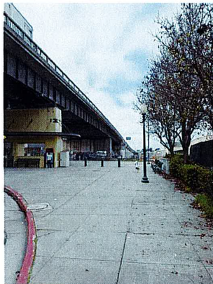
VIEW ALONG UNIVERSITY AVE. TOWARDS WEST
