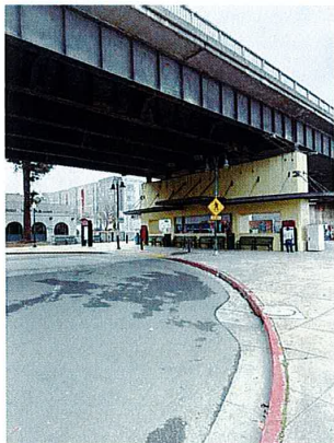
VIEW ALONG UNIVERSITY AVE. TOWARDS WEST
