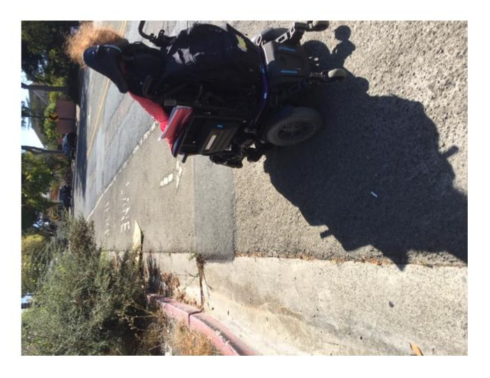
Photo 1: Rose and Henry side uneven tree roots causing cracks and uneven pavement making it unsafe for wheelchair users.
