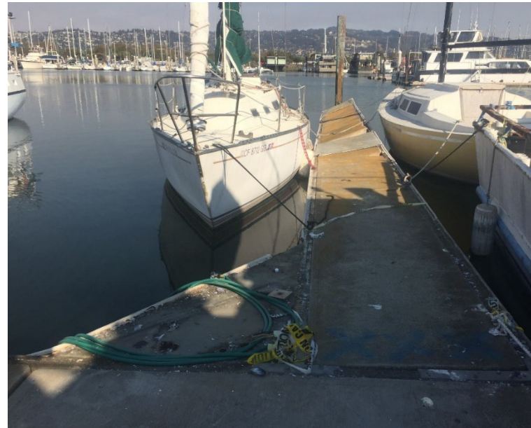
Finger Docks Replacement
