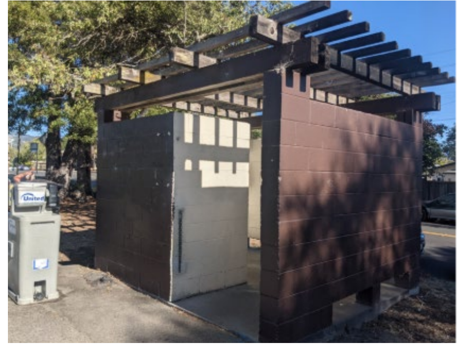
Park Restroom Replacement Project
