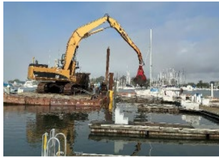
Marina Harbor Dredging
