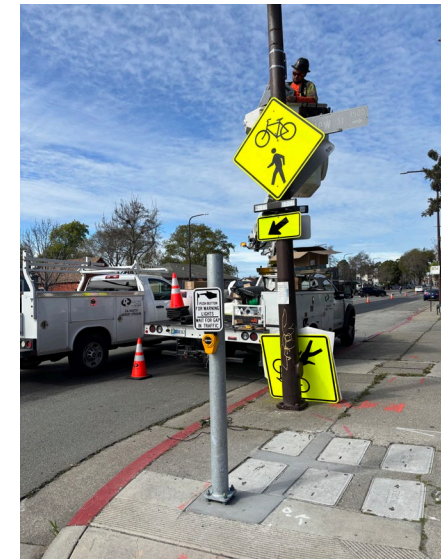
Sacramento Pedestrian Safety Improvements
