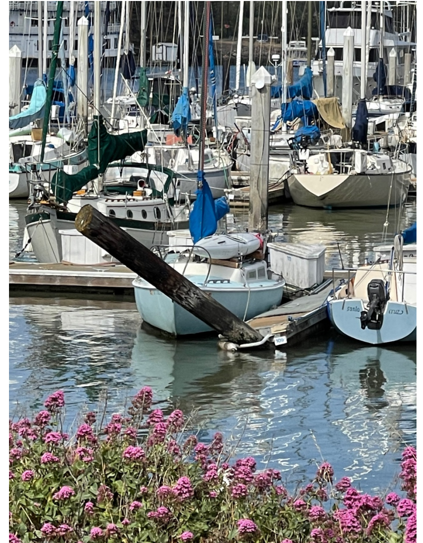
Failed piling
