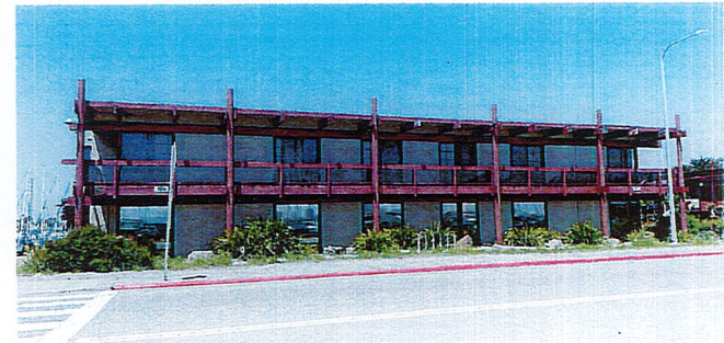
125-127 University Ave. (Office suites & BPD Traffic Bureau)
